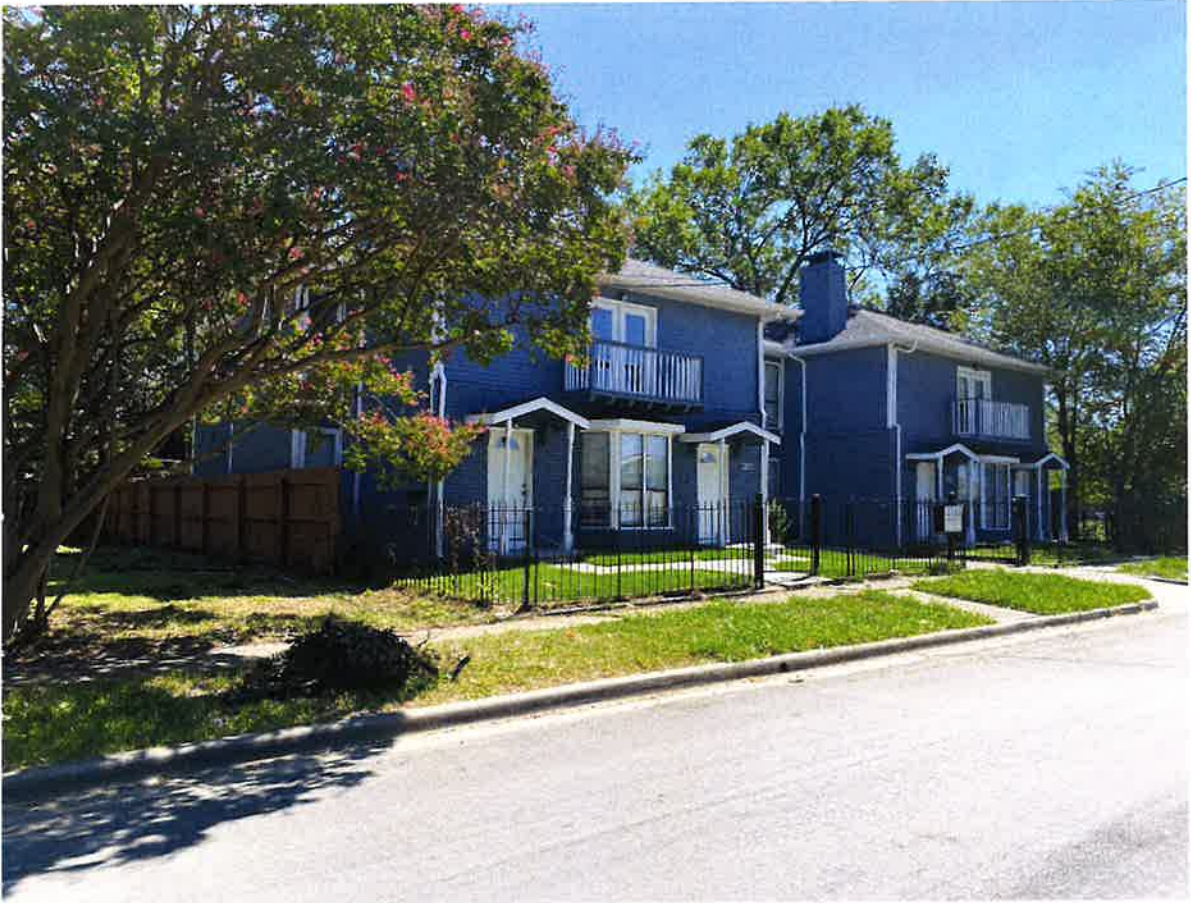
Right (northeast) elevation of duplexes.
