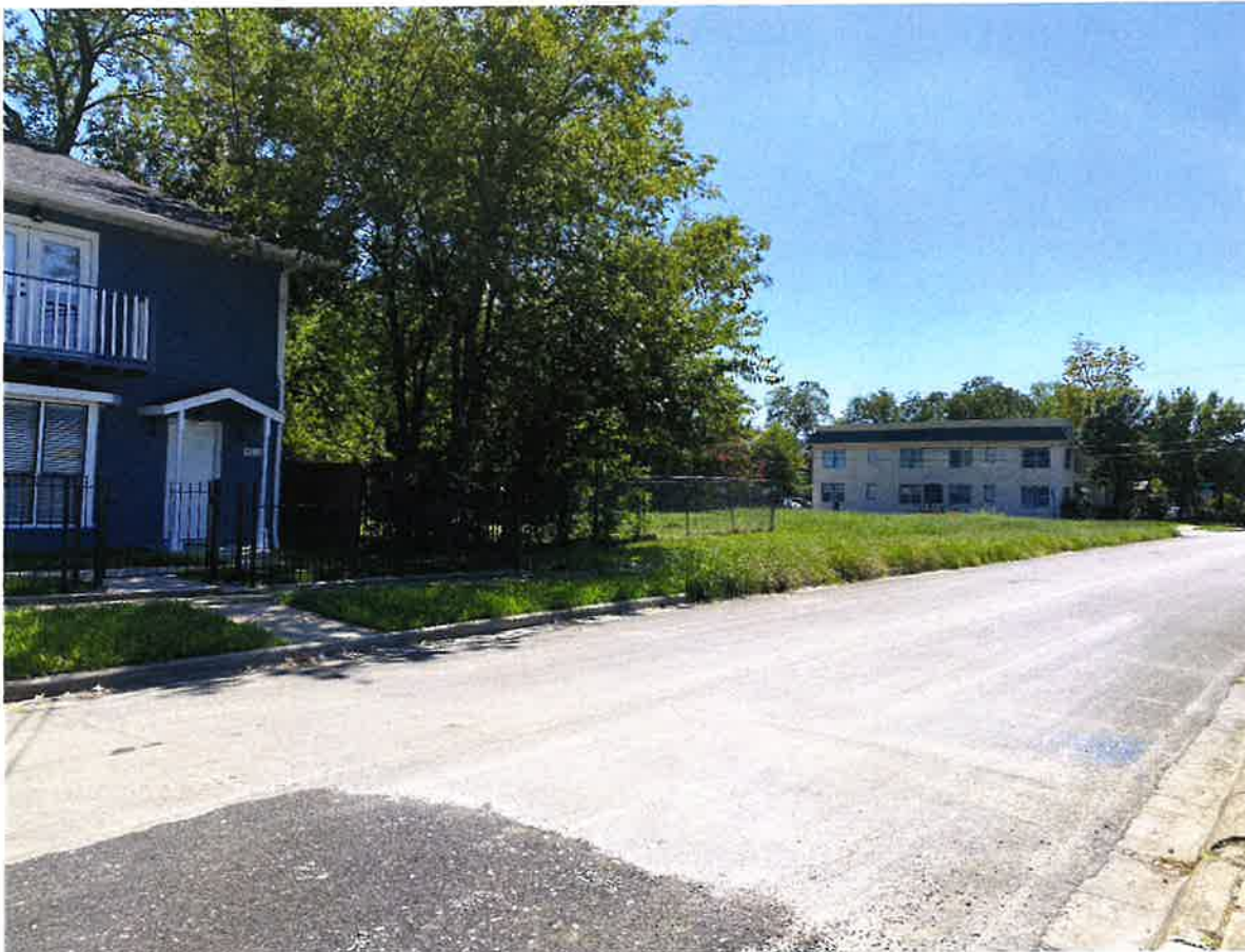
Sycamore St. to the left (direction: southwest) of subject property.
