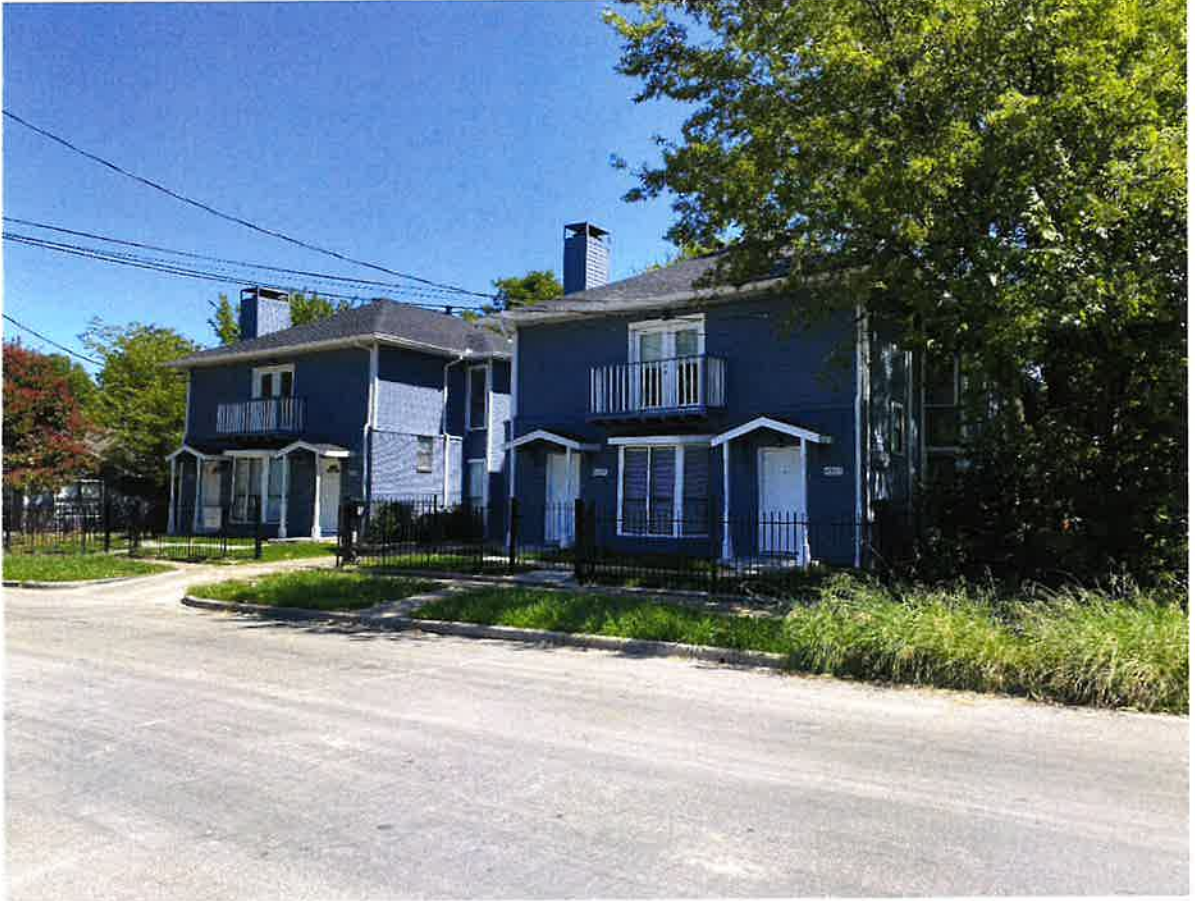
Left (southwest) elevation of duplexes.
