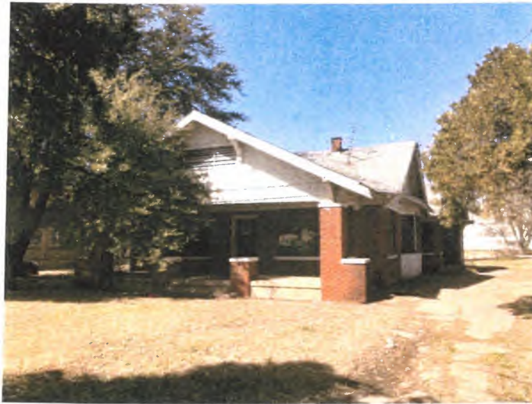
Current Photos: Front view of the structure.
