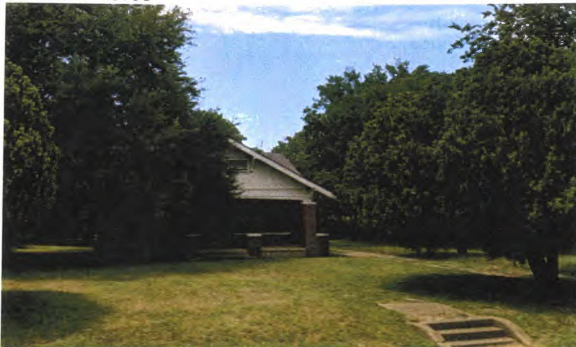
Figure 2. Front View of Main Structure.
