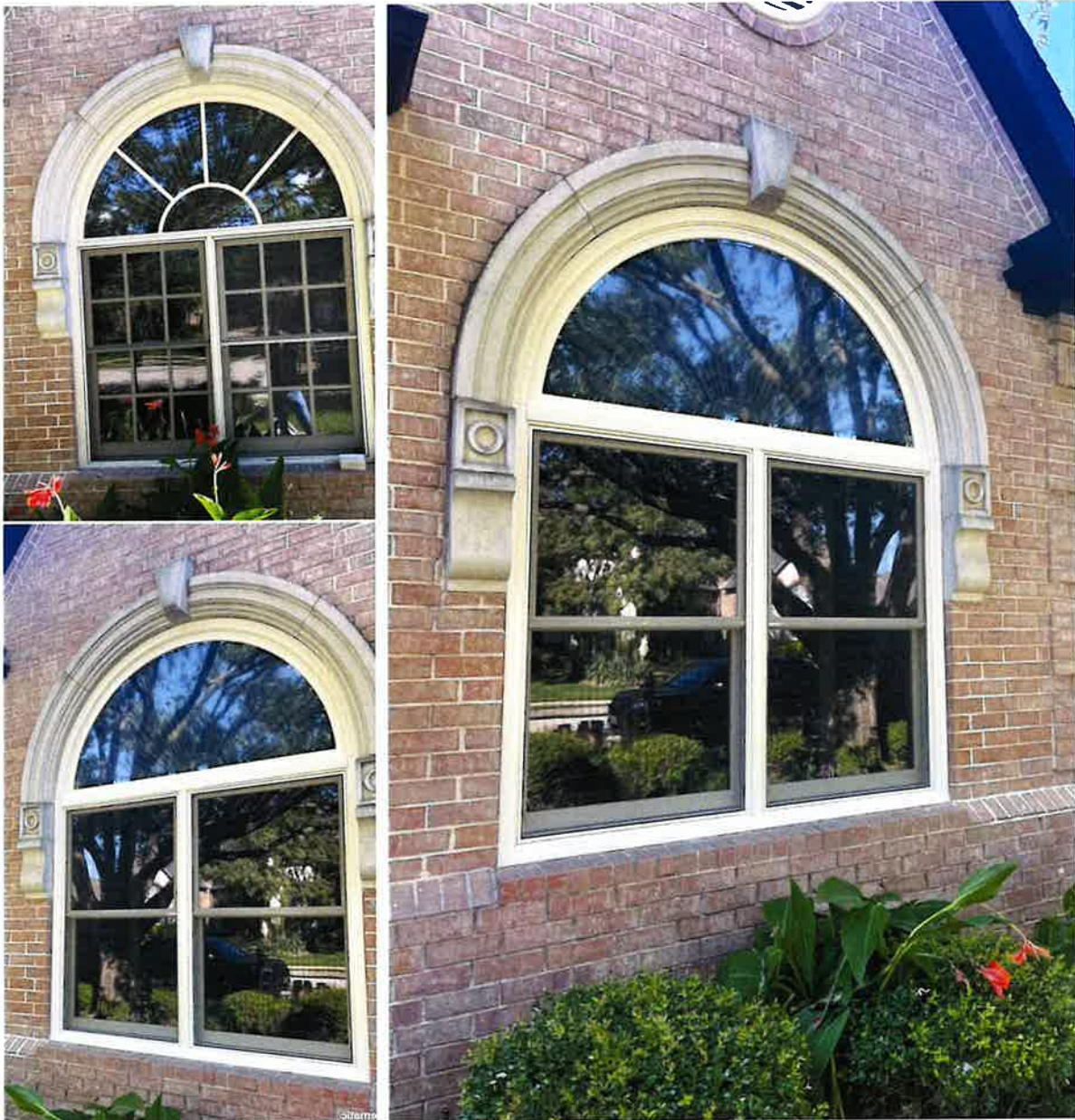
Top: Old window. Bottom: Fibrex® replacement window.
