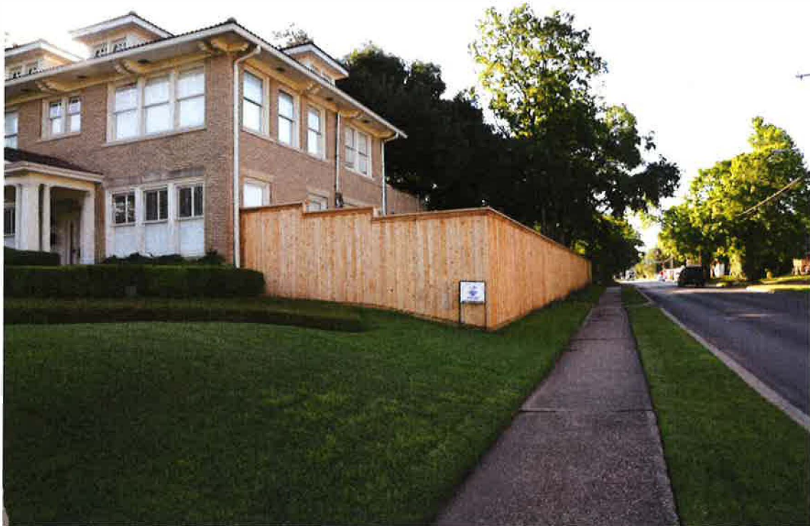
Newly installed fence
