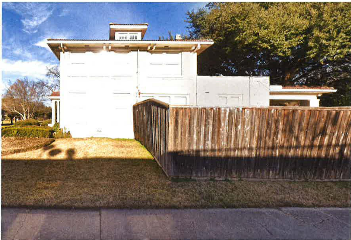
Original fence location
