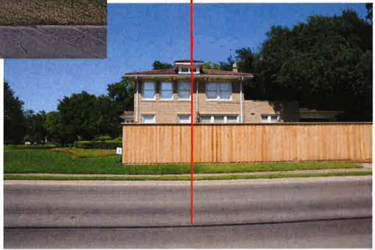
View of new fence from across N Fitzhugh
