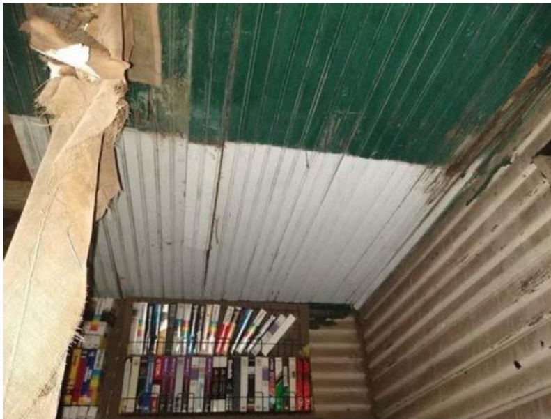
Photo #4. Interior of porch enclosure showing original exterior grade bead-board ceiling. Note the two ceiling paint colors. Originally, there was a wall that divided the bathroom from a screened enclosure between bathroom and side entrance to house.
