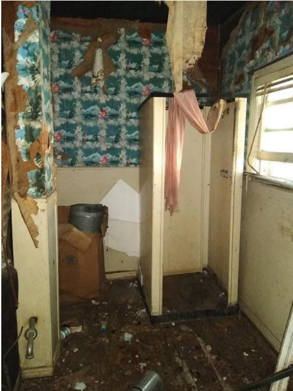
Photo #5. Interior of porch enclosure showing metal shower stall. (Disconnected soon after 1959 due to water leaks.)
