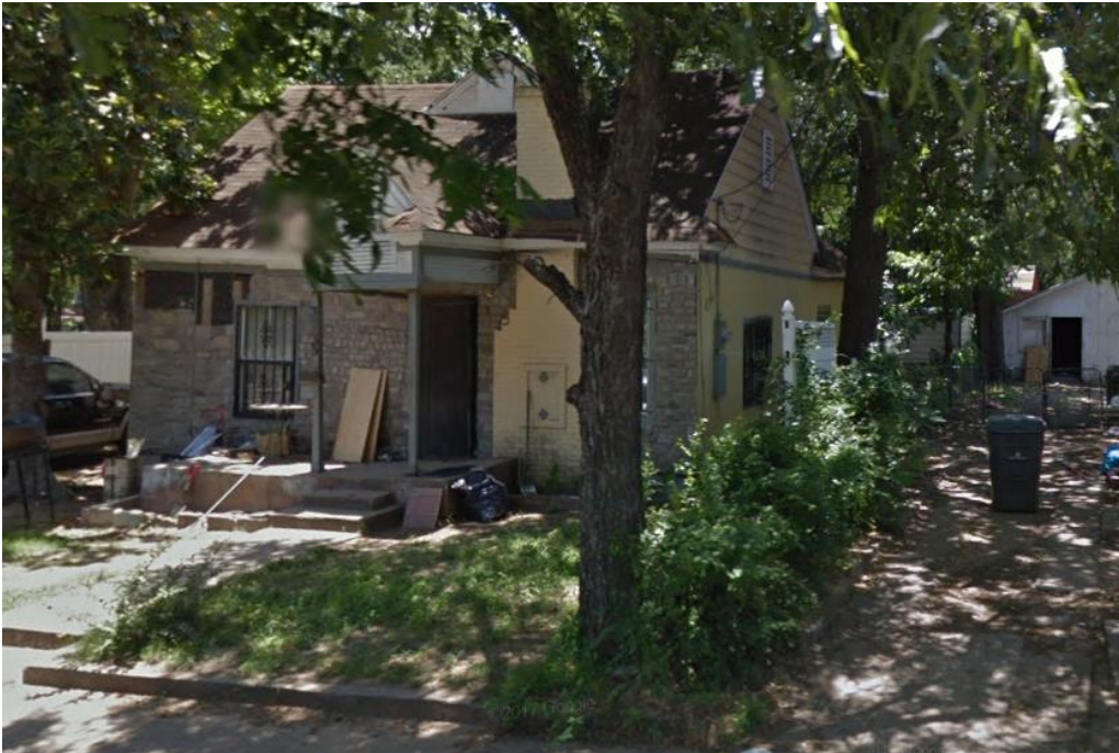
Google image of house, June 2014. Note existence of chimney, brick veneer on front façade, no fan light in front gable, and right front window (just behind tree) that has now been re-located.
