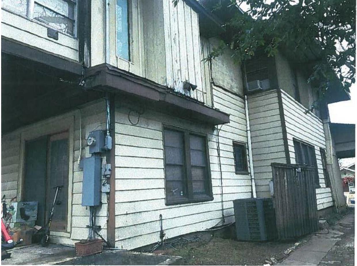
Left (South) and rear elevation. Photo submitted by applicant.
