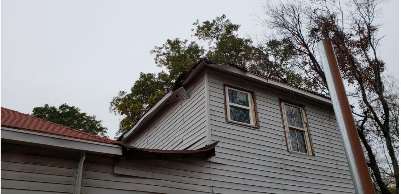
Request #s 2 and 3 – Photo submitted by applicant showing current vinyl siding and cornice.
