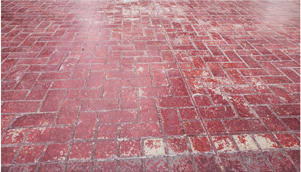
Request #1 – Existing Brick Pavers
