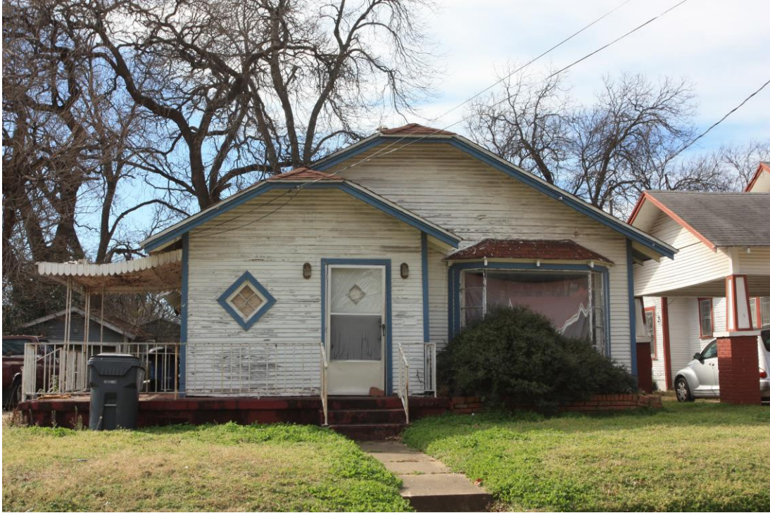
3603 Havana – Example of houses in Wheatley Place with small stoop and no porch.
