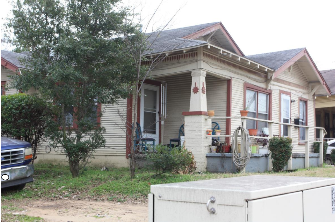
View to right (West) of 2826 Metropolitan.
