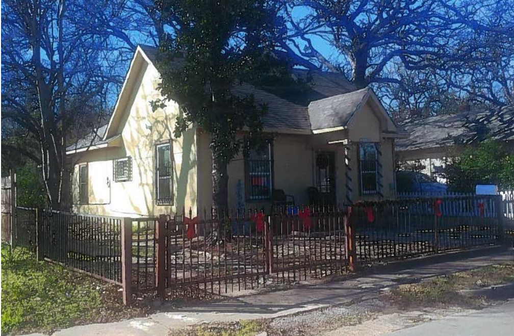
Left (South) side elevation. Photo submitted by applicant.
