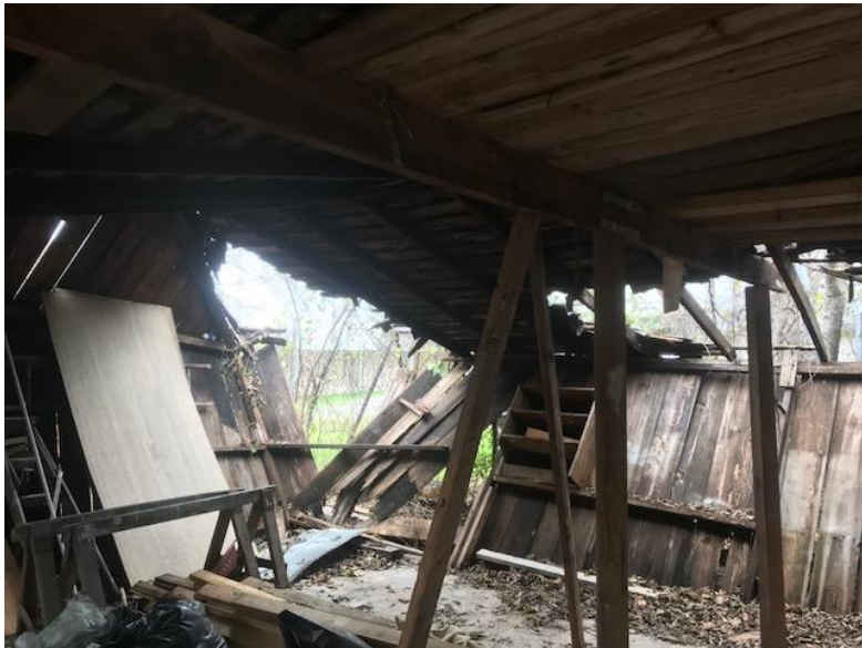
Existing conditions of accessory structure
