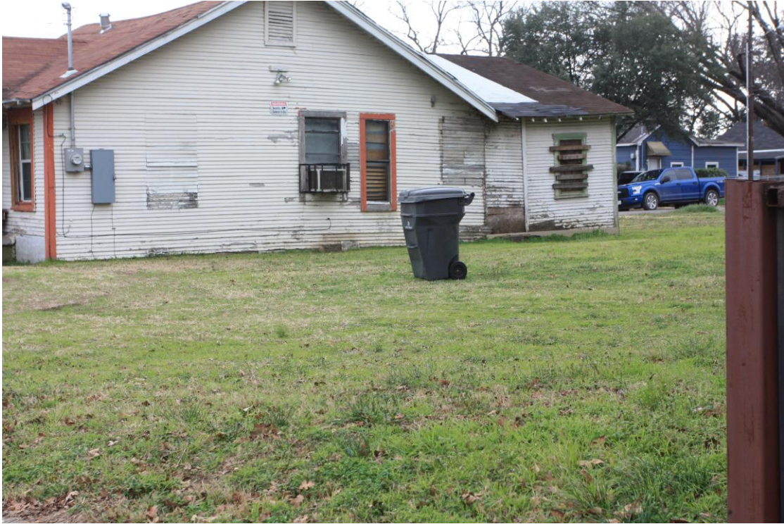
View to left (South) of 3735 Havana.
