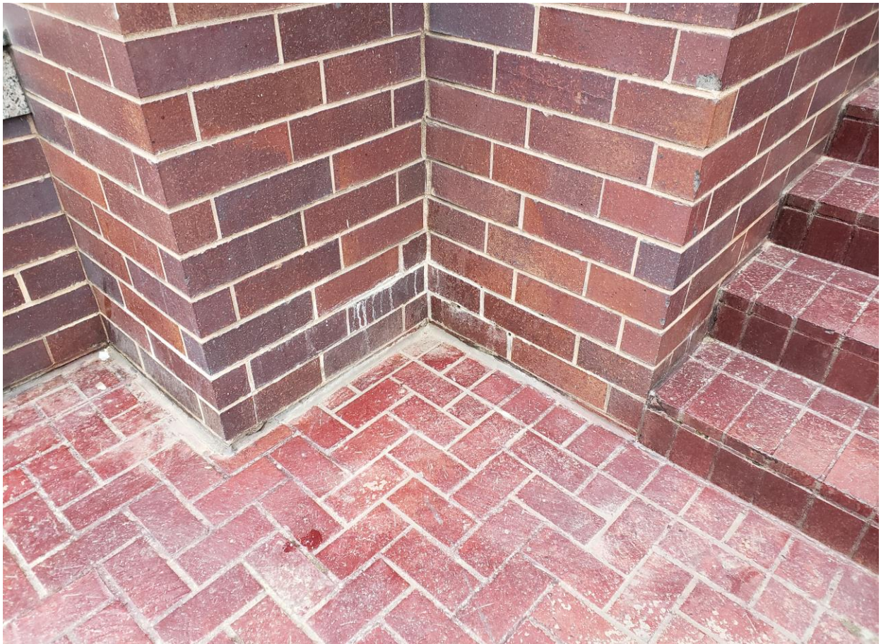
Request #1 – Existing Brick Pavers (note contrast between pavers and building/planter cladding)
