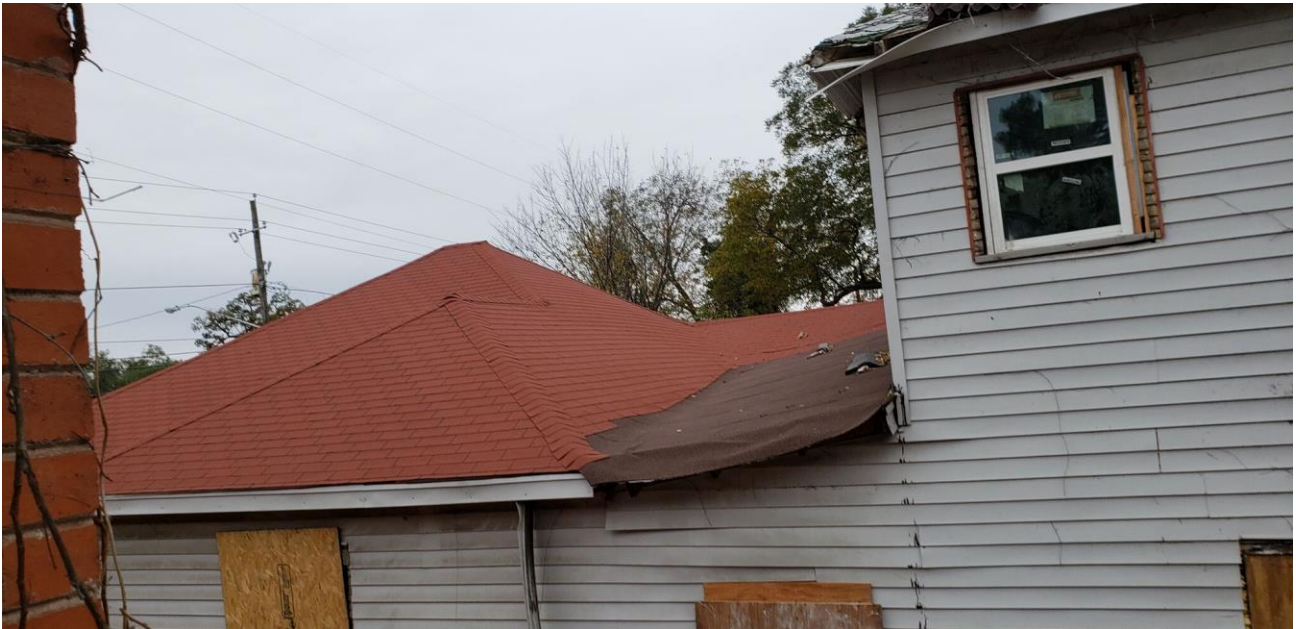
Request #s 2 and 3 – Photo submitted by applicant showing current vinyl siding and cornice.
