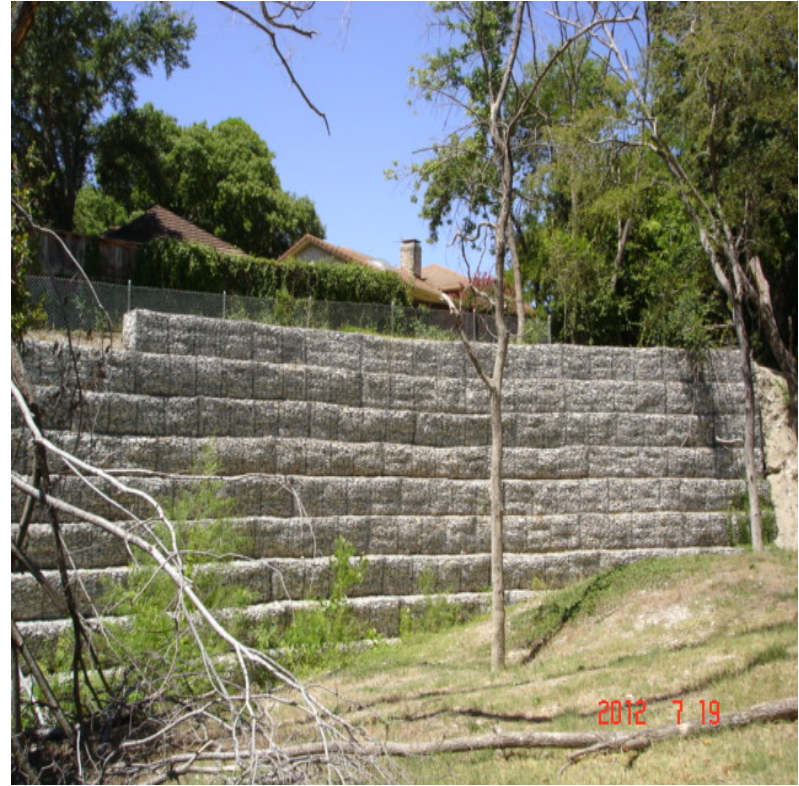
9539 Rocky Branch Drive Construction Completed (2012)
