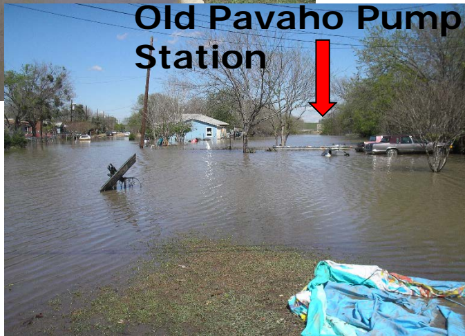
West Dallas Area South of Canada Drive Before Pavaho Pump Station (2006)
