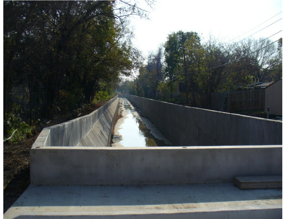
Elam Creek Phase I After construction (2012)
