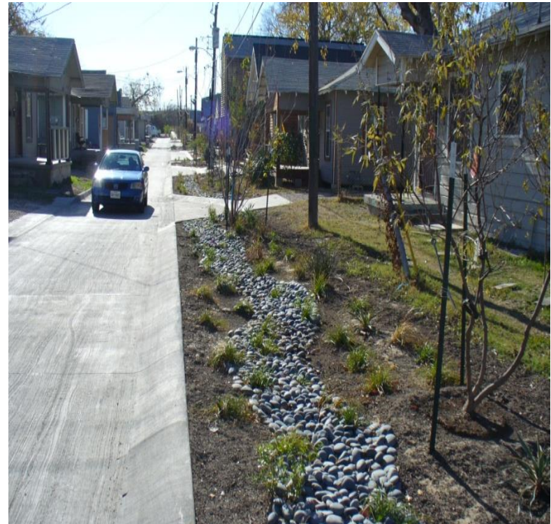
Bioswale and landscaping
