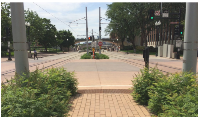
This light-rail platform leads to a large crosswalk that is paved with a different, distinguishable material
