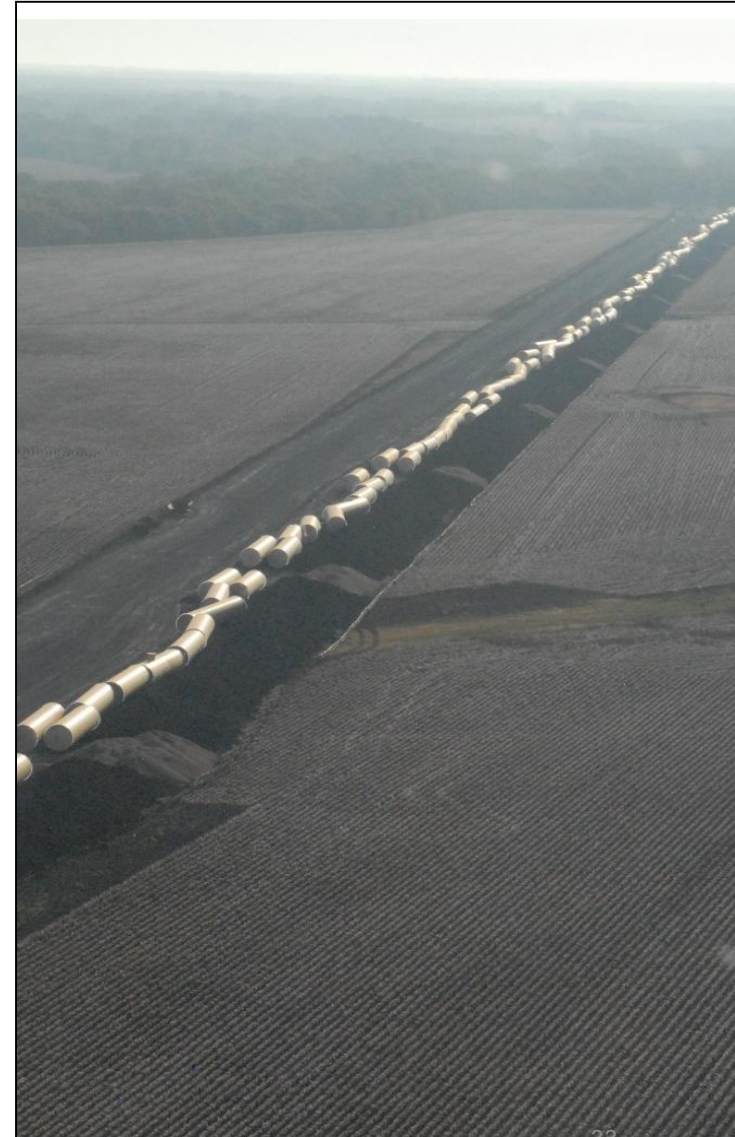
Pipe for Segment 15-2 in Ellis County
