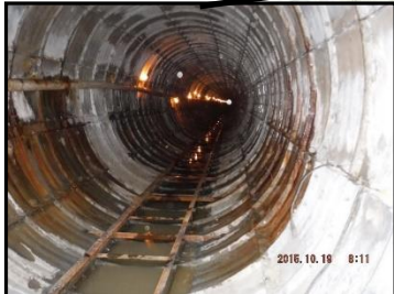
Tunnel under US 67 in Midlothian
