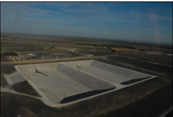
JB3 Pump Station Suction Reservoir
