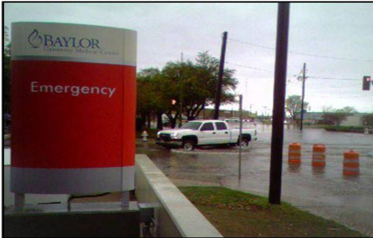
Flooding of part of Baylor Hospital facilities on March 19, 2006
