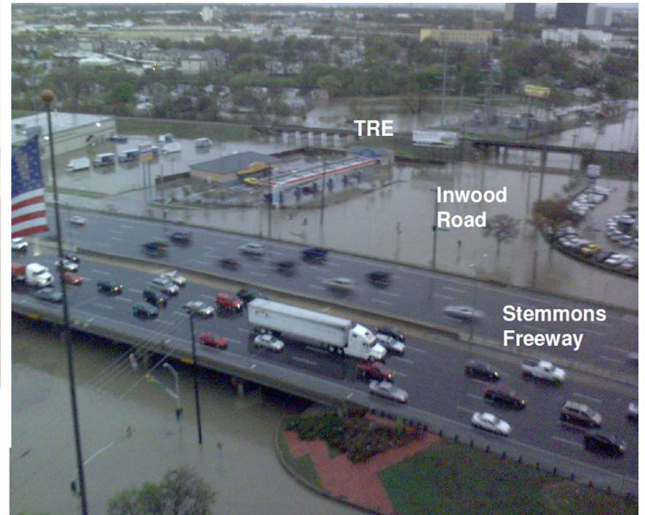
Photo 3.7 - Inwood Road at Stemmons Freeway (IH35E), Record Crossing Sump Area - March 19, 2006
