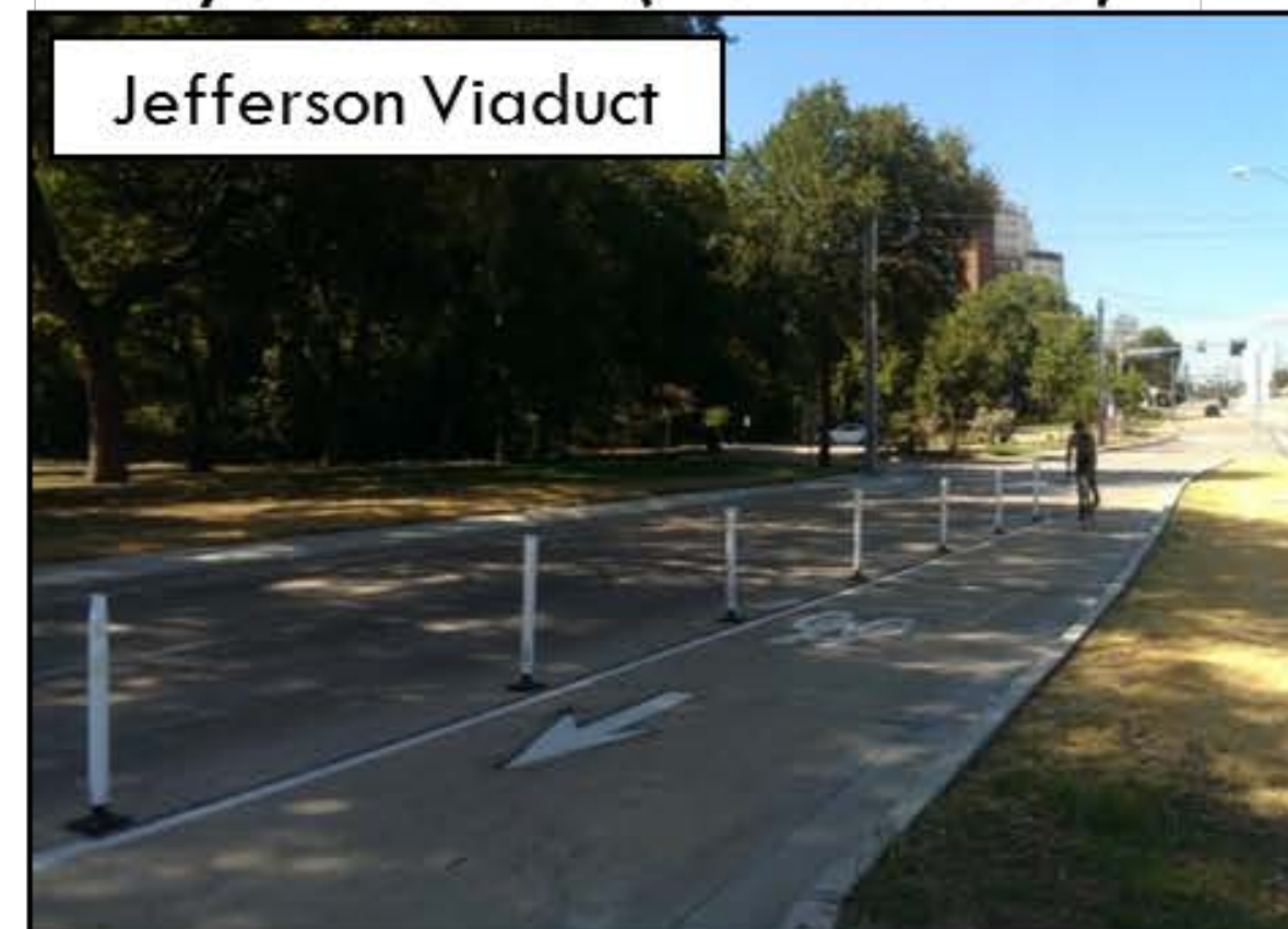
Physically Separated Bicycle Lanes (flex stakes)
