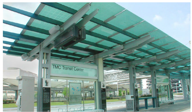
This station platform has a large and shaded canopy, seating, wayfinding, and historical education elements
