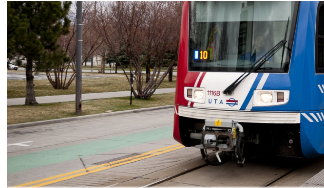
This light rail has rumble strips adjacent to the tracks to warn motorists not to enter the lane
