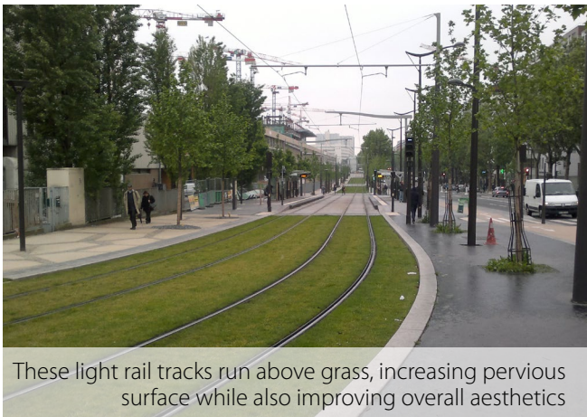
Landscaping beneath the tracks and along the tracks is preferred due to aesthetics and stormwater management
