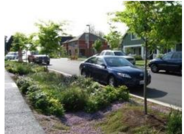
A bioswale and permeable concrete are used for stormwater management and to enhance neighborhood aesthetics (Source: Abby Hall, US EPA)
