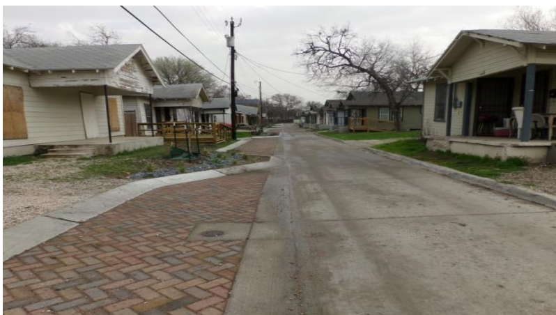
Permeable pavement in recessed parking areas
