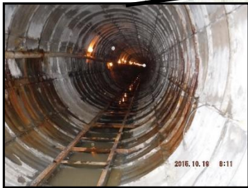
Tunnel under US 67 in Midlothian
