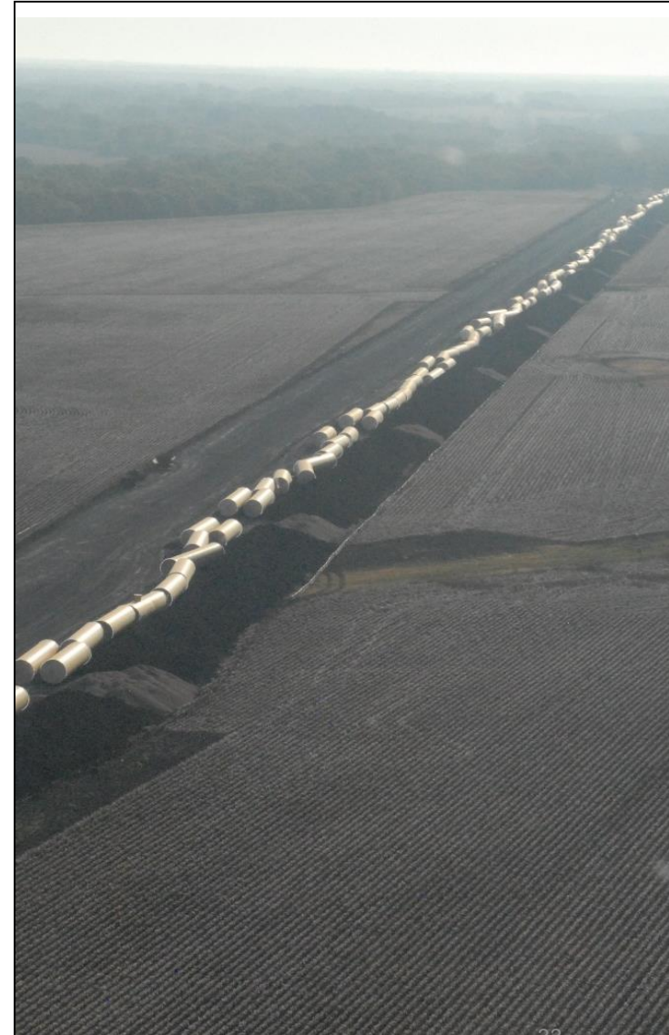
Pipe for Segment 15-2 in Ellis County
