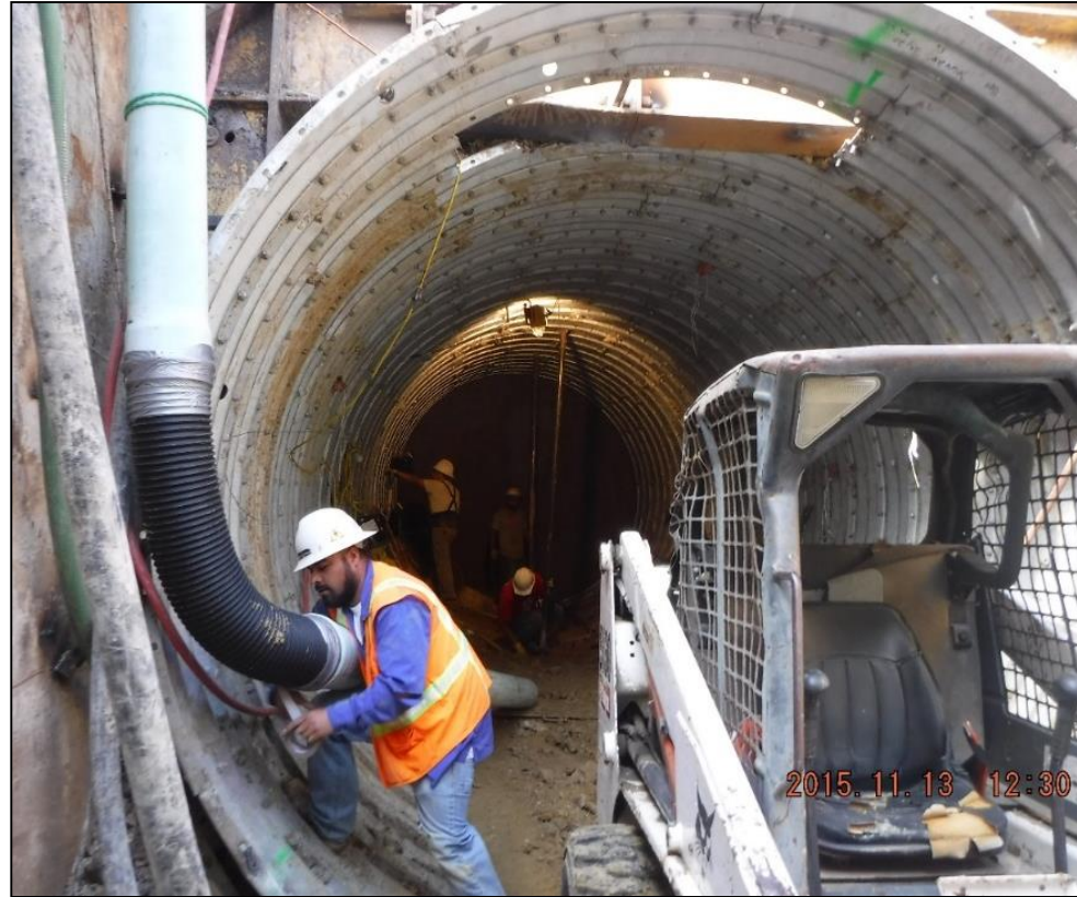
Tunnel under Farm to Market 985 near Lake Bardwell in Ellis County
