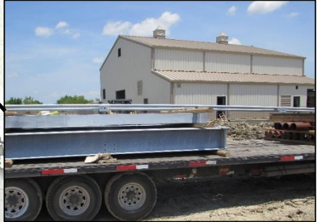
Richland Chambers Interconnect Facility
