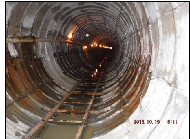
Tunnel under US 67 in Midlothian
