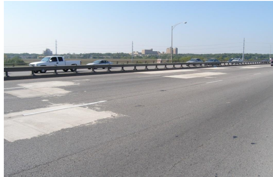
I-30 Bridge Deck Repairs
