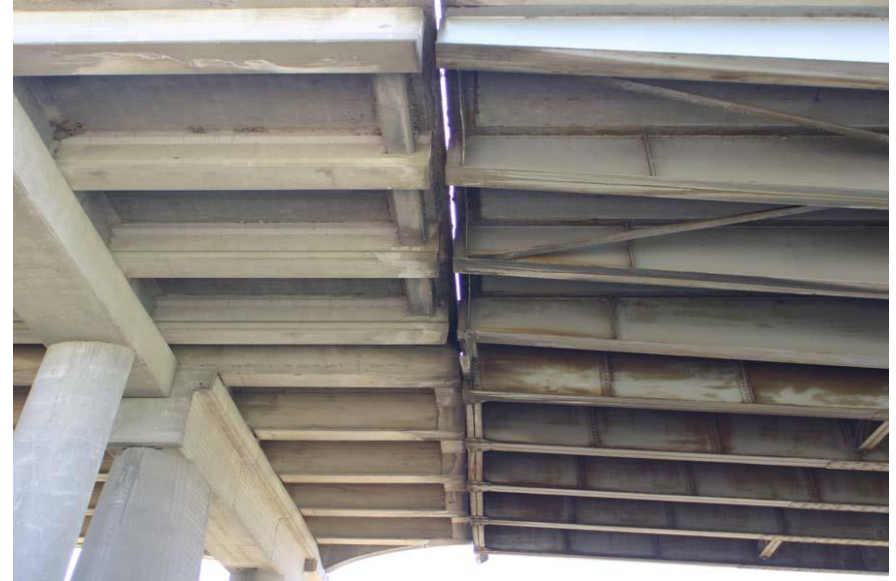
I-35E Bridge Joint at Main Span
