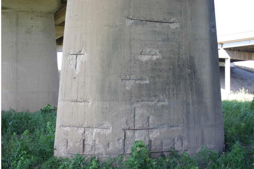
I-35E Bridge Substructure
