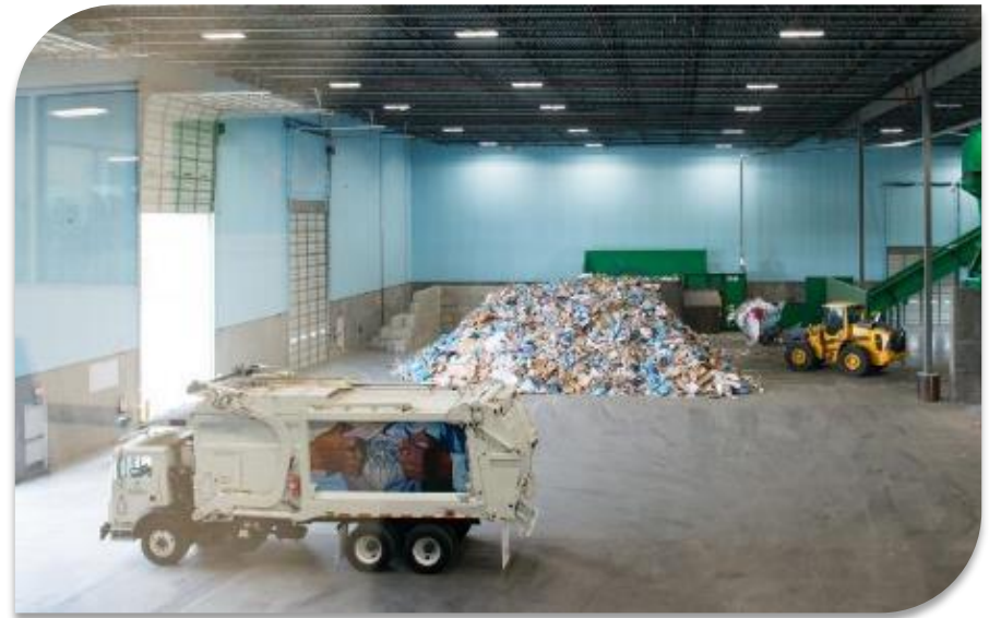
Tipping Floor View From Gallery
