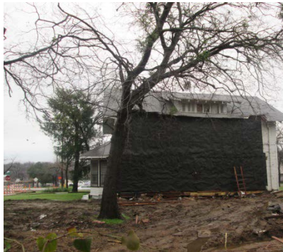
Decaying & Damaged TREES
