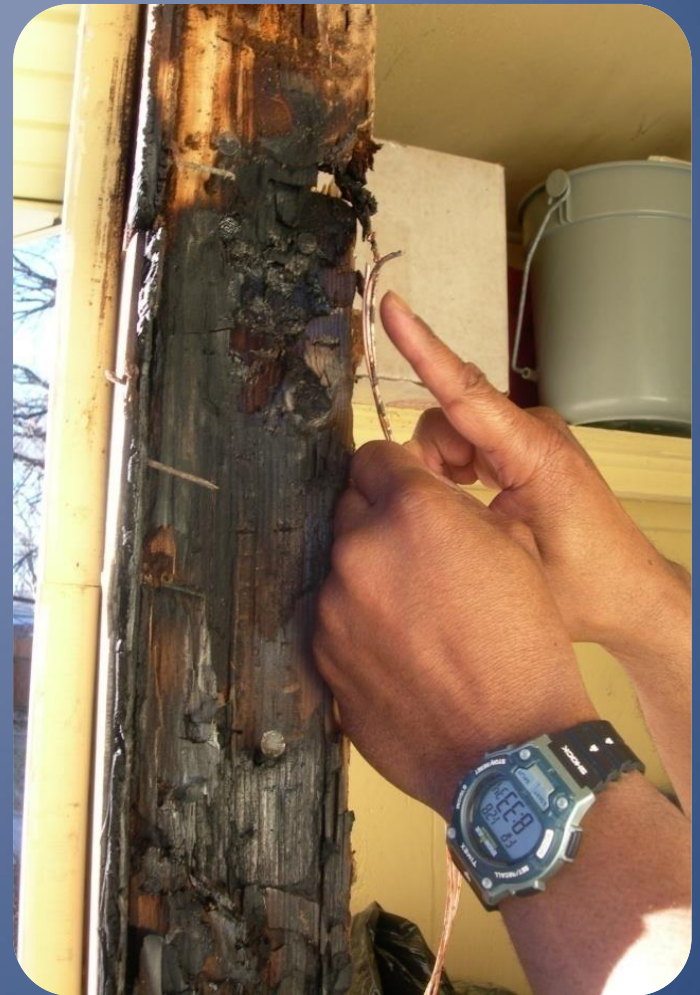
Electrical Failure
