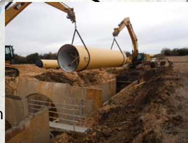
Installation of 108-inch pipe along Section 17
