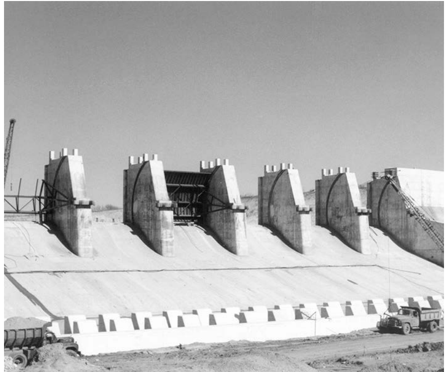
Forney Dam at Lake Ray Hubbard Installation of Tainter Gates
