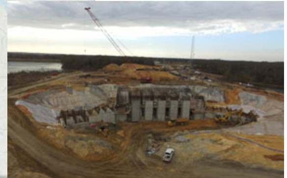
JB3 Pump Station Suction Reservoir
