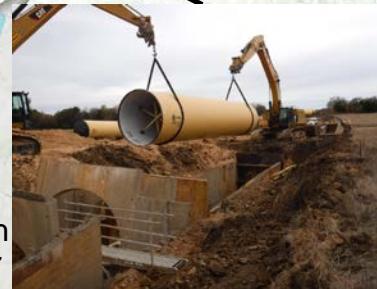
Installation of 108-inch pipe along Section 17
