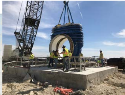
108-inch Gate Valve Installation
