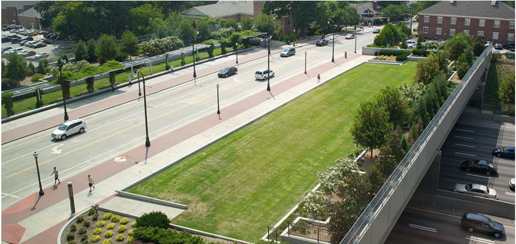
Example – Atlanta Fifth Street Bridge
