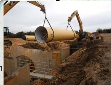
Installation of 108-inch pipe along Section 17
