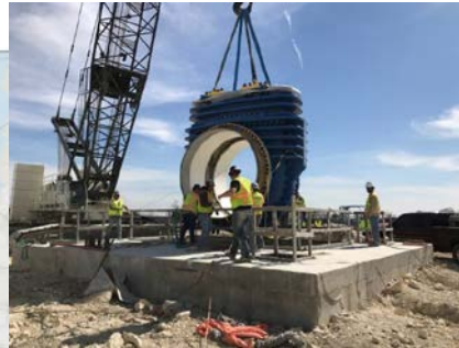
108-inch Gate Valve Installation
