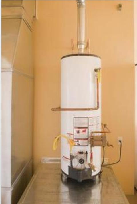
Hot water heaters are required to have a pressure relief valve to prevent the water tank from exploding. The valve is mounted either on the top or side of the tank and must extend to the outside of the structure. The pipe must extend to the exterior of the structure.
