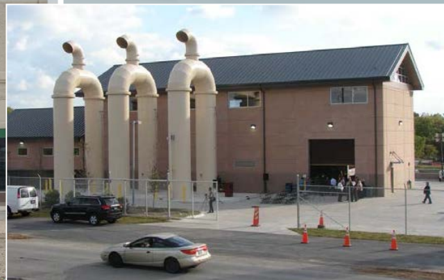
Pavaho Pump Station
