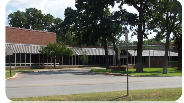
Bachman Recreation Center $3.9M
