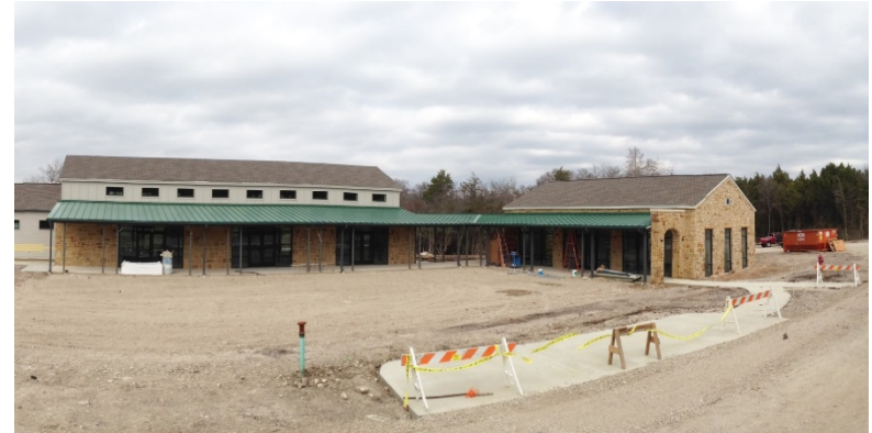
The Rees-Jones Foundation Welcome Center Complex
