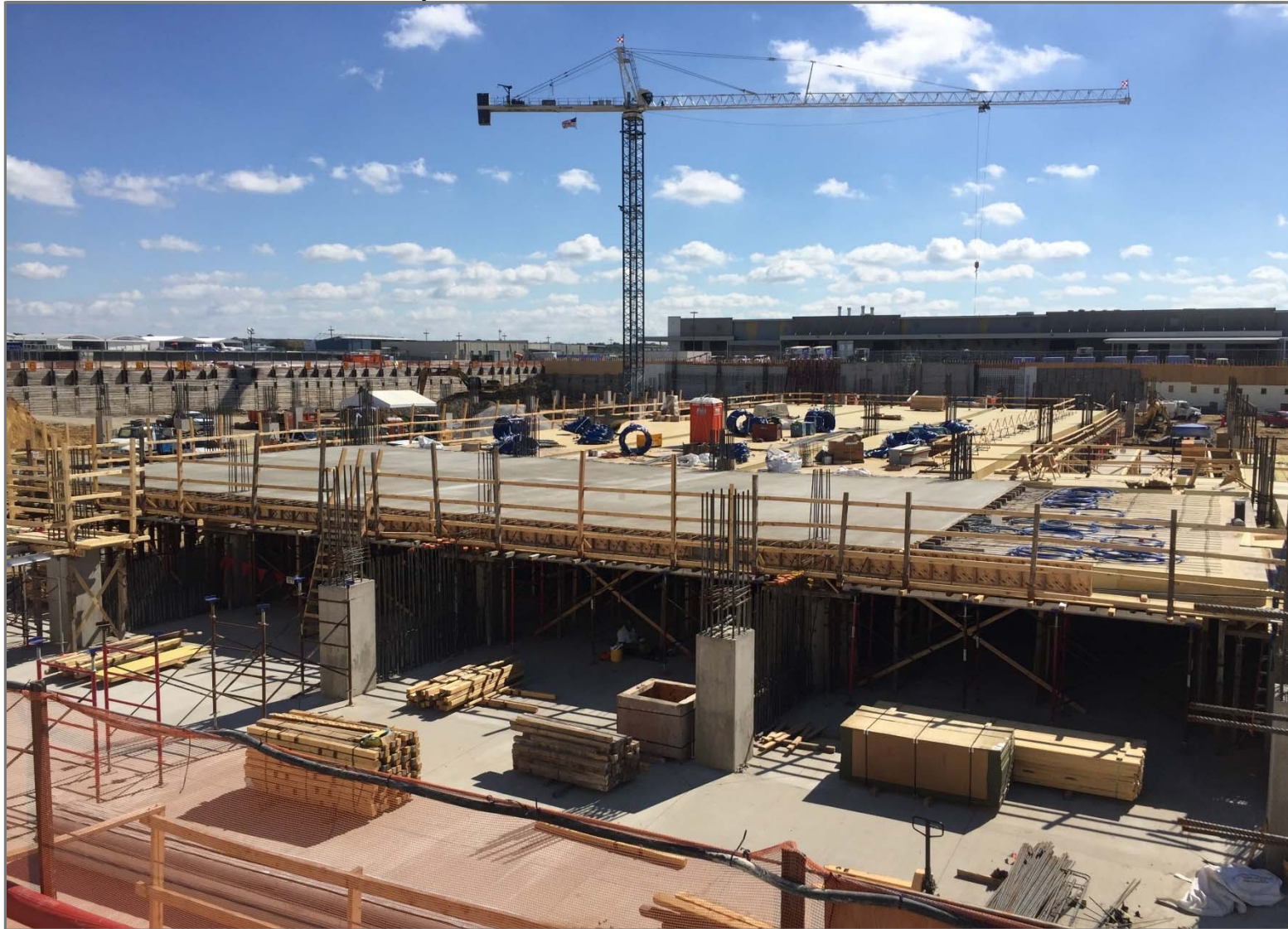
Level 1 deck concrete placement
