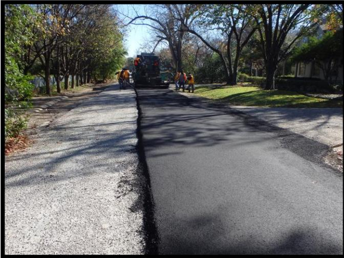
**Rehabilitation** - A treatment for ASPHALT STREETS when a large portion of the surface and the base have deteriorated to an unsatisfactory level. It includes the full-depth repair of base failures, followed by a chip seal, and a new two-inch layer of hot mix asphalt placed over the entire treated segment. Candidate streets are predominately residential asphalt surfaced streets without curb and gutter. **Cost:** \$150K per lane-mile. **Life:** 10-12 years.
