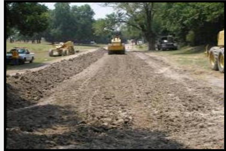
**Restoration** - A treatment for ASPHALT STREETS when the entire surface and the base have deteriorated to an unsatisfactory level. It includes rebuilding the entire base by recycling the old base and surface materials into a new base, followed by a chip seal, and new two-inch layer of hot mix asphalt placed over the entire treated segment. Candidate streets are predominately residential asphalt surfaced streets without curb and gutter. **Cost:** \$164K per lane-mile. **Life:** 18-20 years.
