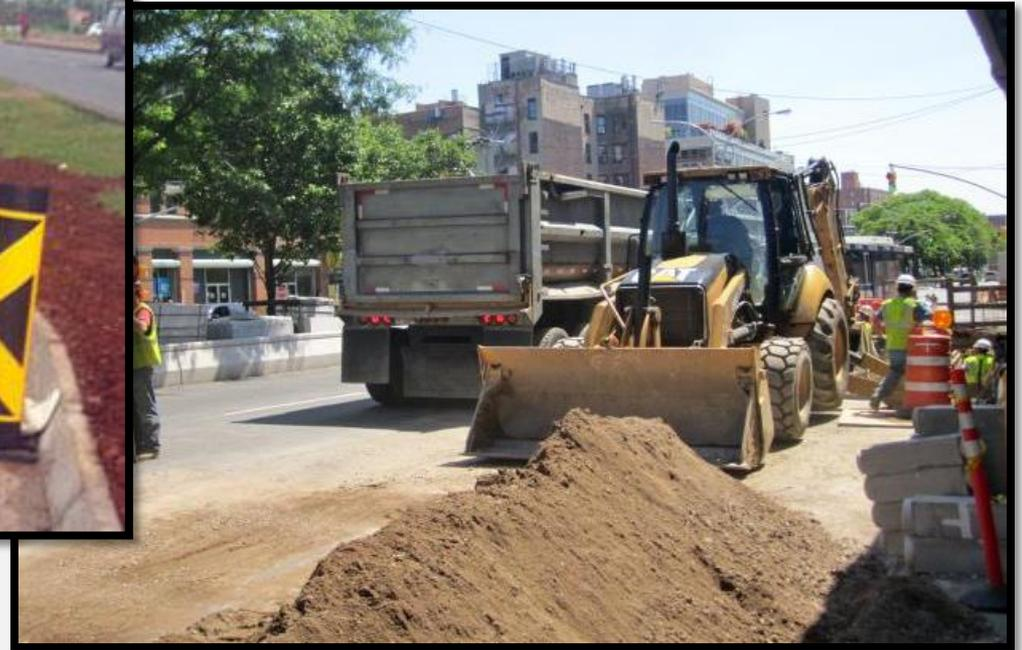
Street and alley repairs by the Dallas Water Utilities are associated with pipeline replacement. For asphalt streets the City policy requires that an entire lane be reconstructed at the location for where the pipeline is replaced. From joint to joint for concrete streets.
