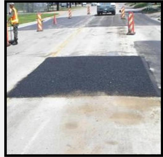
**Slurry Seal** - This treatment for CONCRETE STREETS WITH ASPHALT SURFACE consists of a ¼-inch layer of sand and fine stone mixed with asphalt emulsion. This seals and smooths the surface and conceals scars from previous repairs. It is used predominately for residential roads with curb and gutter. The work is outsourced to a specialized contractor – after Street Services performs preparation work (such as minor base repair and crack sealing).
