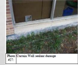
Photo #27: Curtain Wall sealant damage
