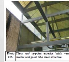
Photo #36: Clean and re-point exterior brick veneer; mortar and paint masonry structure
