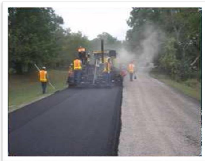
Asphalt Street Overlay (Rehabilitation)
