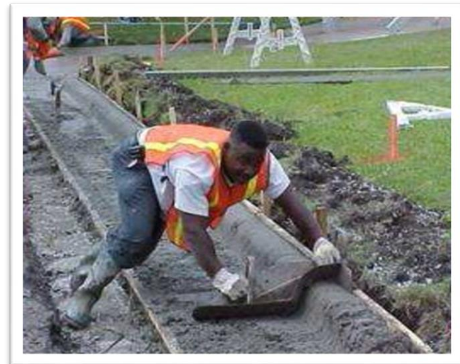
Concrete Curb and Gutter
