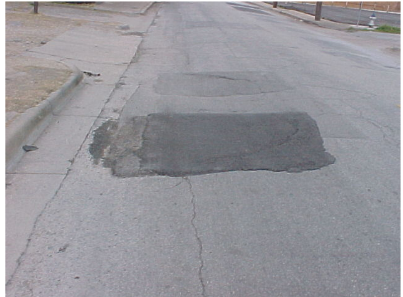
Temporary Repair to Asphalt Street
