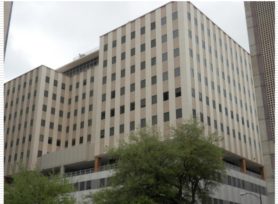
Continental Building – South/West Side
