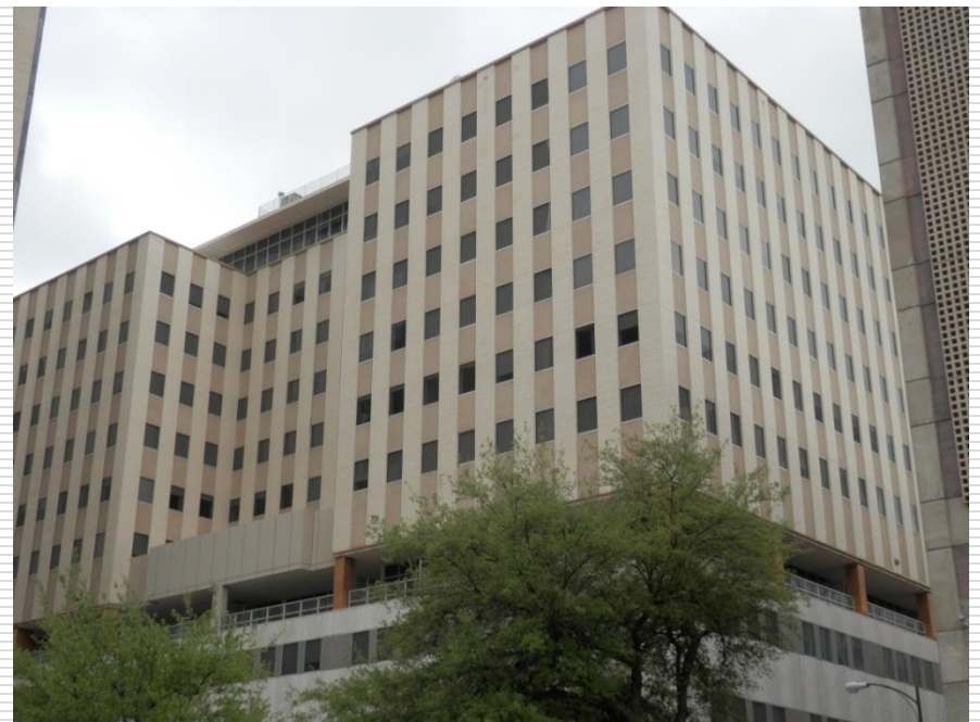
Continental Building – South/West Side
