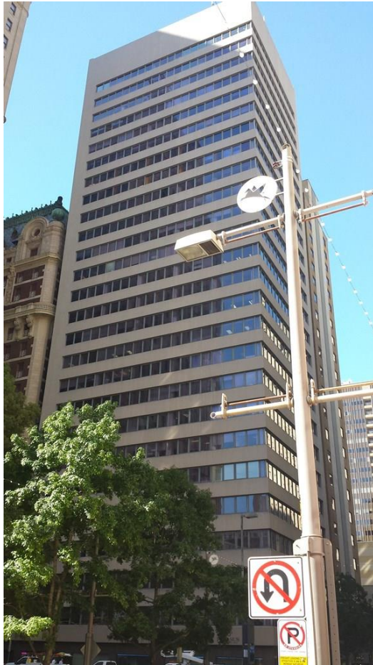
1412 Main Street Corrigan/Adolphus Tower 1954 Current Owner: BN 1412 Main LP Retail/Office
