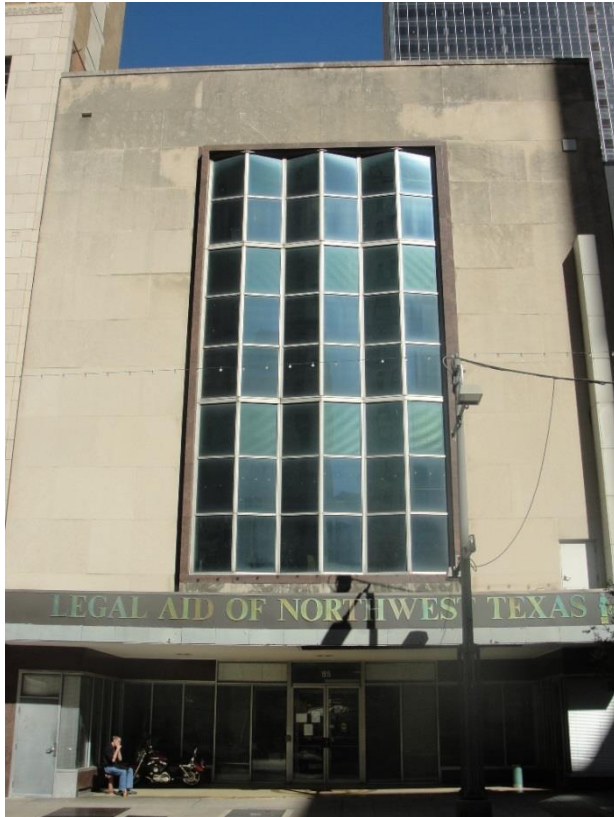
1515 Main Street Jas K. Wilson Building 1947 Current Owner: Legal Aid of Northwest TE Office
