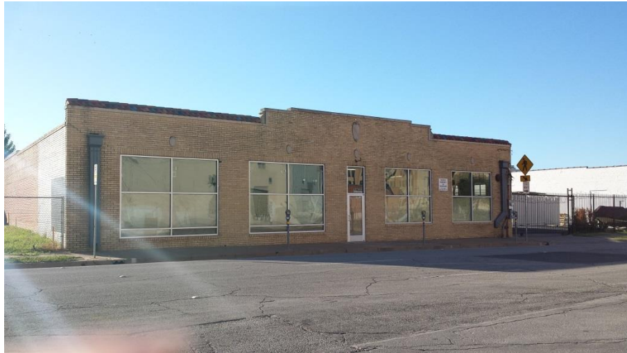
1820 Canton Street One story commercial structure 1930 Current Owner: Salamander Group LLC
