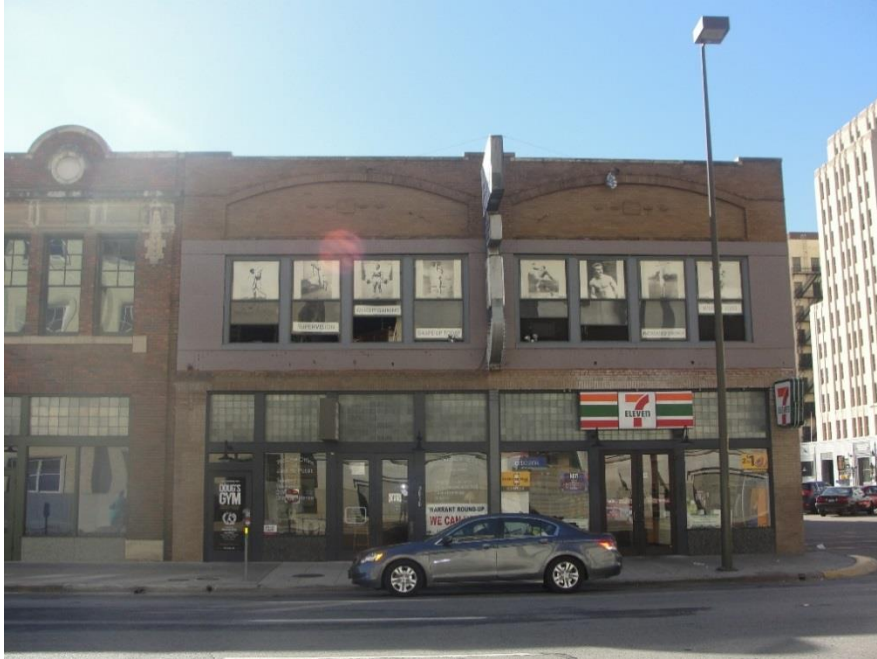
2008-2010 Commerce Street Doug's Gym/7-11 c. 1910 Current Owner: ASC Harcom Investments Retail
