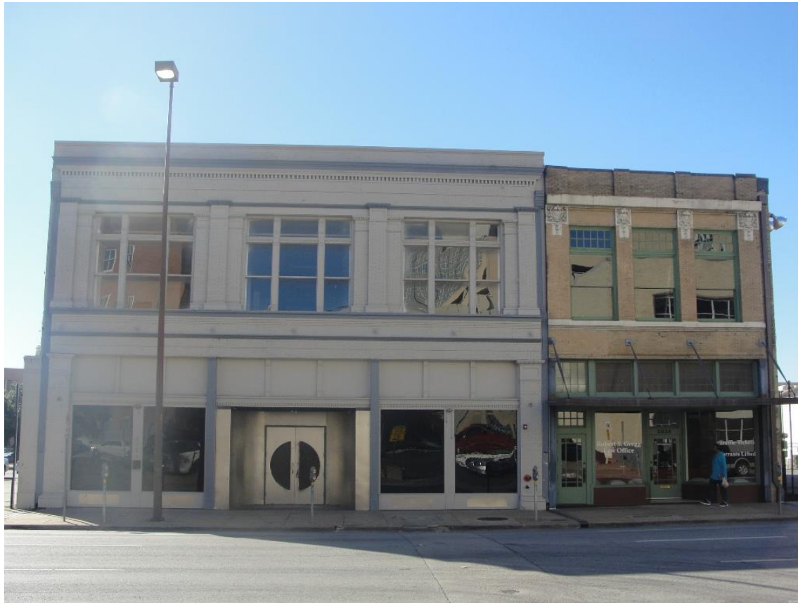
2026 Commerce Street Two-story commercial building c. 1915 Current Owner: CADG 2026 Commerce LLC Vacant
