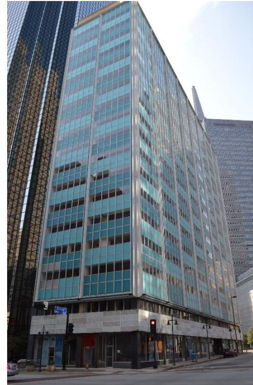
211 N Ervay 1958 Current Owner: Alterra 211 North Ervay LLC Office/retail – under construction City Center TIF ($2,000,000)
