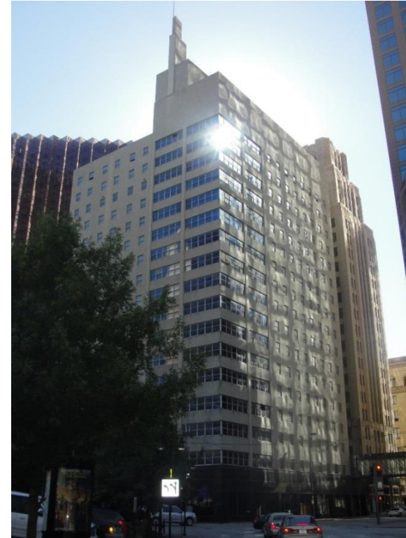
1900 Pacific Street Corrigan Tower 1952 Current Owner: PetroCorrigan Towers LP Vacant – future construction Downtown Connection TIF ($10,300,000 allocated*)
