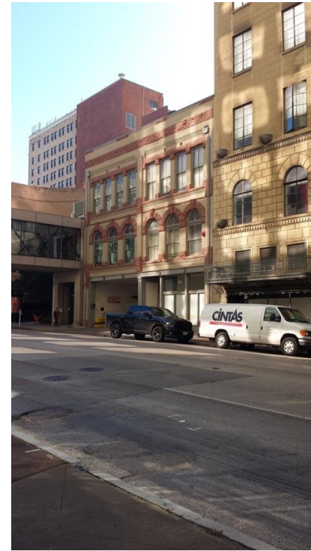
1908 Elm Street Titcher Annex 1902 Current Owner: Jarvis Barney W Jr TR & Mary Lou TR Residential City Center TIF and Federal Tax credit
