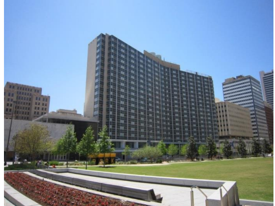
1914 Commerce Street Statler Hilton Hotel 1956 Current Owner: Commerce Statler Development LLC Vacant – under construction Downtown Connection TIF ($46,500,000 - combined with Old Public Library) and Pending Federal Tax Credit – Future construction
