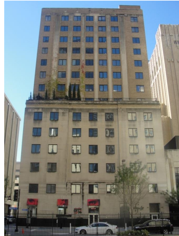
1512 Commerce Street Continental Supply/Texaco Building 1903 (later additions) Current Owner: DPL Loans Holdings LLC Residential/retail City Center TIF and Federal Tax credit
