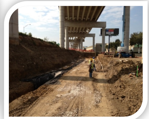
BRIDGE 7C AND MSE WALL 4 SB LOOP 12
