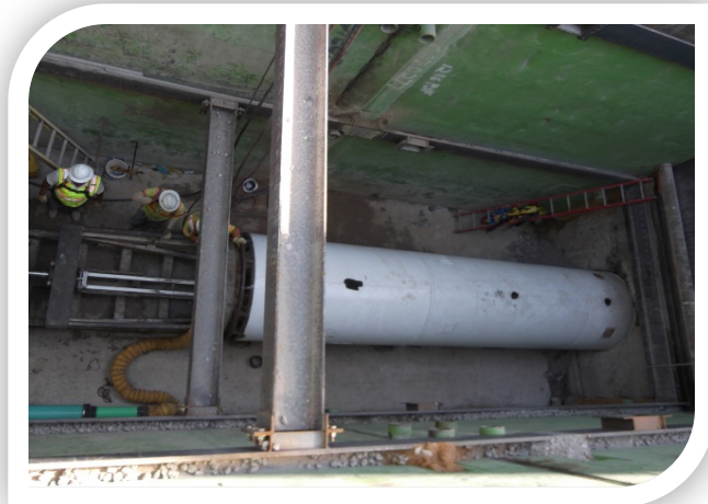
JACK & BORE FOR DEEP DRAINAGE AT MANAGED LANES
