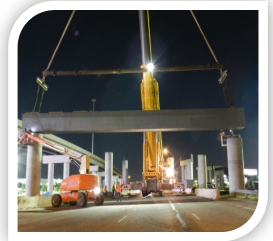
STEEL CAPS NB IH 35 MANANA EXIT
