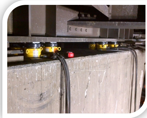
JACKING OPERATION AT INWOOD BRIDGE
