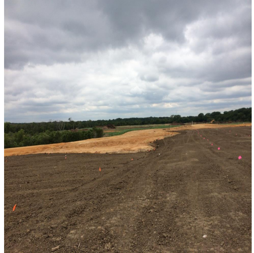
Cap Repair with Clay & Vegetative Support
