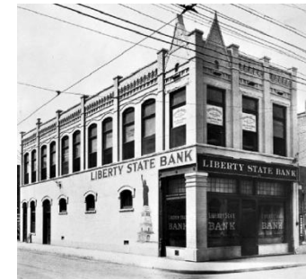
Liberty State Building Relocation
