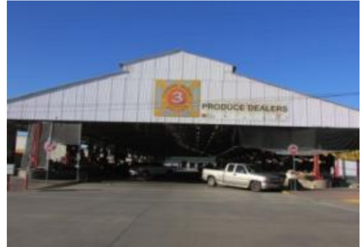
Existing Shed 3 picture
