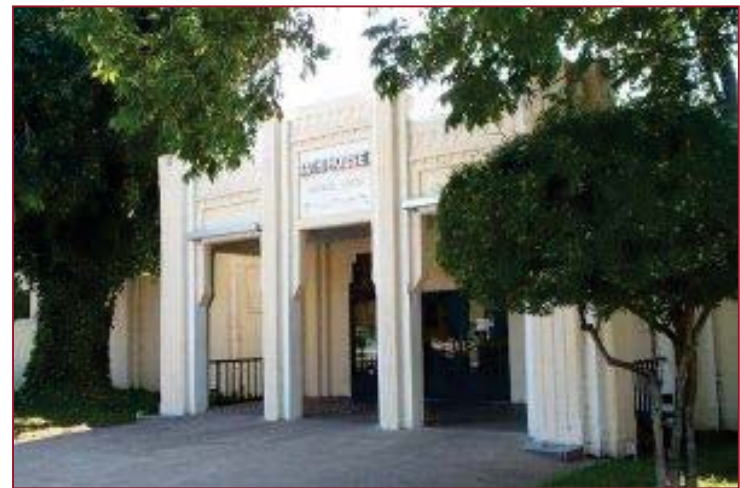
BHCC exterior view
