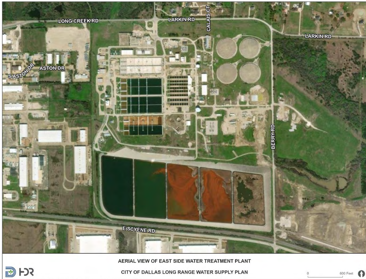
Figure 8-4. Aerial View of the East Side WTP
