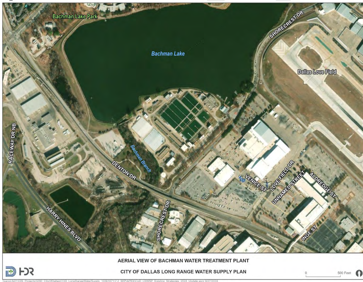
Figure 8-2. Aerial View of the Bachman WTP
