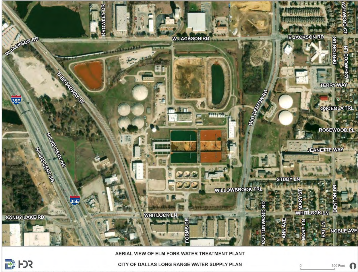
Figure 8-3. Aerial View of the Elm Fork WTP
