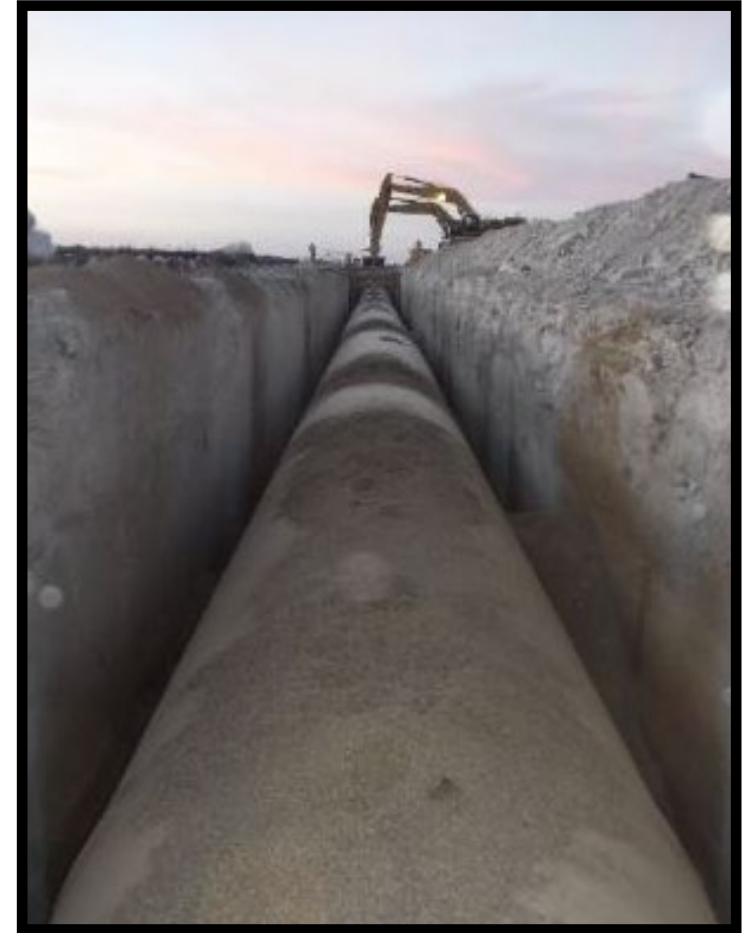
Installation of 108-inch pipe along IPL Section 17
