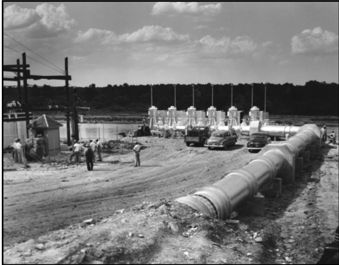
City of Dallas Red River Pump Station, 1953-1957
