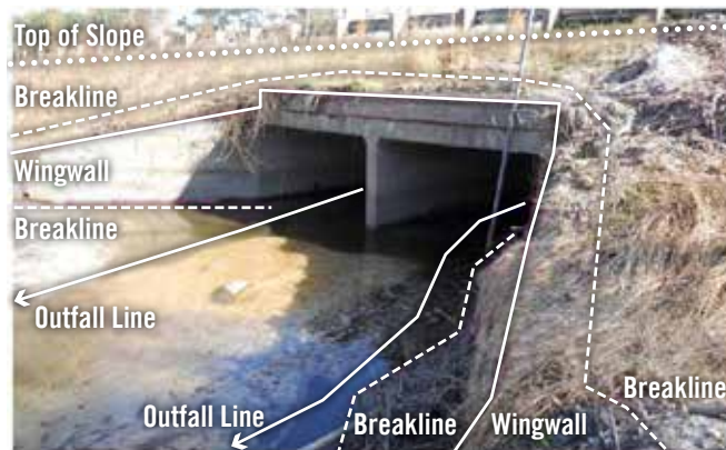
Figure 10.7 Culvert Survey Example
