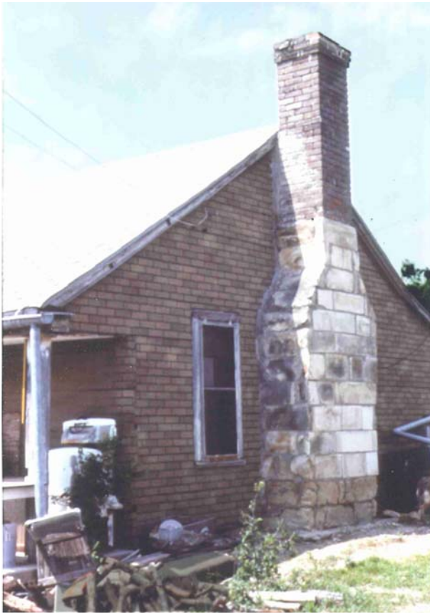
Figure 24 - Farmhouse, north façade showing dressed stone chimney and detail of dressed stone with graffiti in 1976. Note name 'E M Hale' – was the property owner of site from 1894 - 1909. These stones with graffiti are no longer at chimney.
