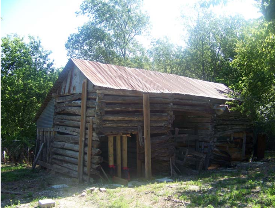
TX_Dallas County_ Everard Sharrock Jr. Farmstead_0004.tif Log Barn Southwest Oblique. Camera facing: Northeast
