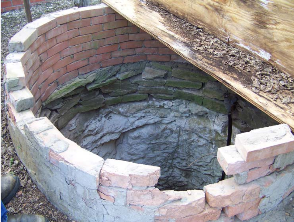
TX_Dallas County_Everard Sharrock Jr. Farmstead_0008.tif Hand Dug Well. Camera facing: South
