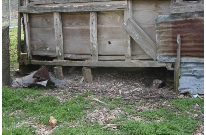
Figure 9 - Log barn – details of crib with bois d’Arc piers, February 2008
