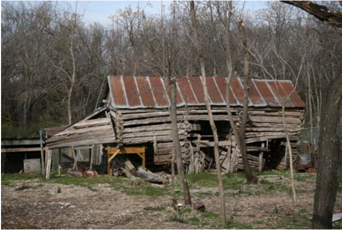
Figure 8 - Overall view of the log barn with lean-to at left, February 2008
