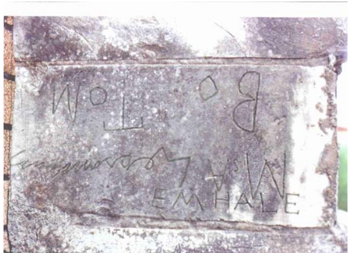
Niblo Chimney dressd limestone block #43, in situ, Feb. 20, 1976 Overlay tracing with enhanced rendering of inoised graffiti
