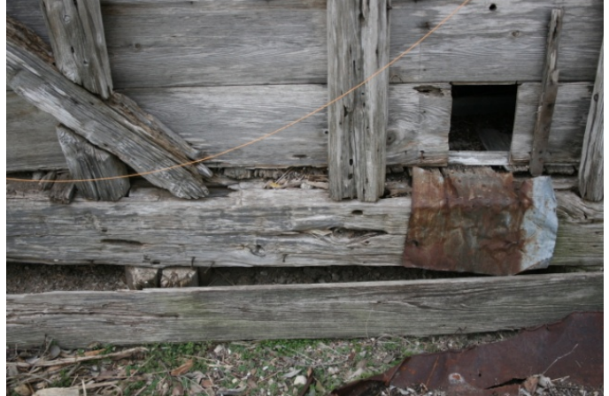
Figure 11 - Log barn foundation at crib, with slot for grain access, February 2008
