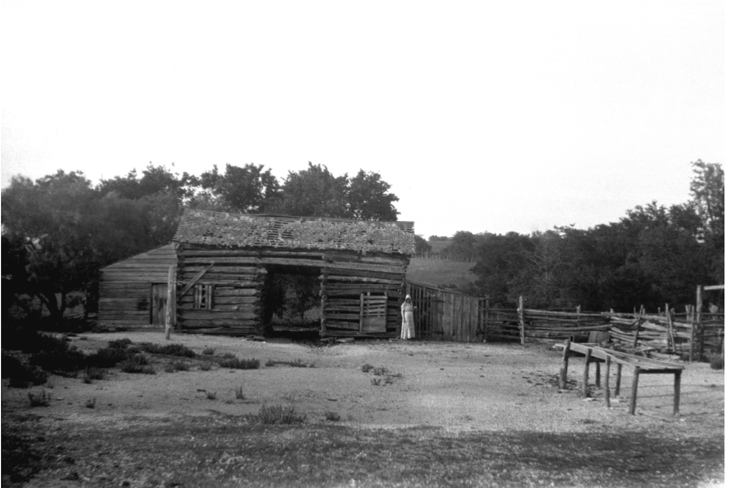
Figure 7 - Log barn, ca. 1934 Photo courtesy of the Niblo Family
