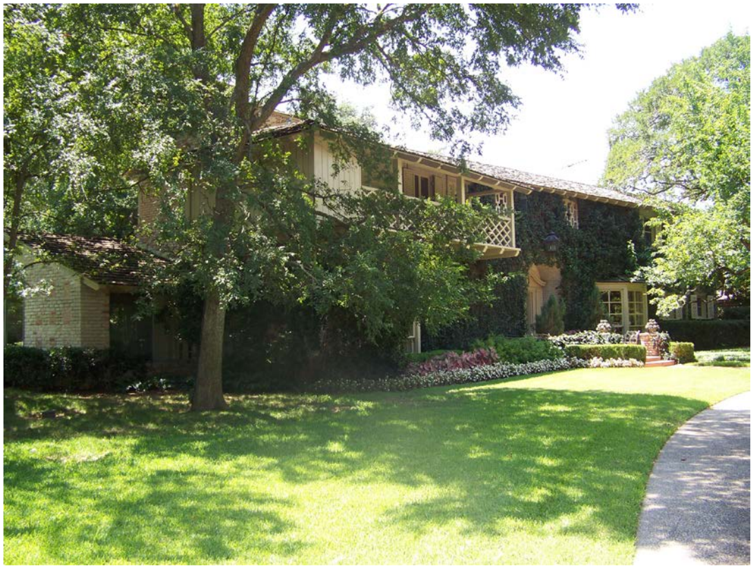
Front elevation with balcony at left. Photographer: Nancy McCoy
