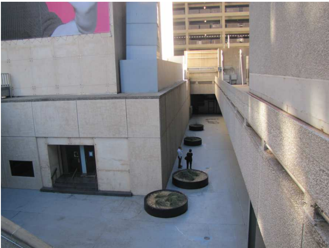
Detail of stair in east sunken-plaza from the southwest (top), October 2014 View into the east sunken-plaza from the north (bottom), October 2014
