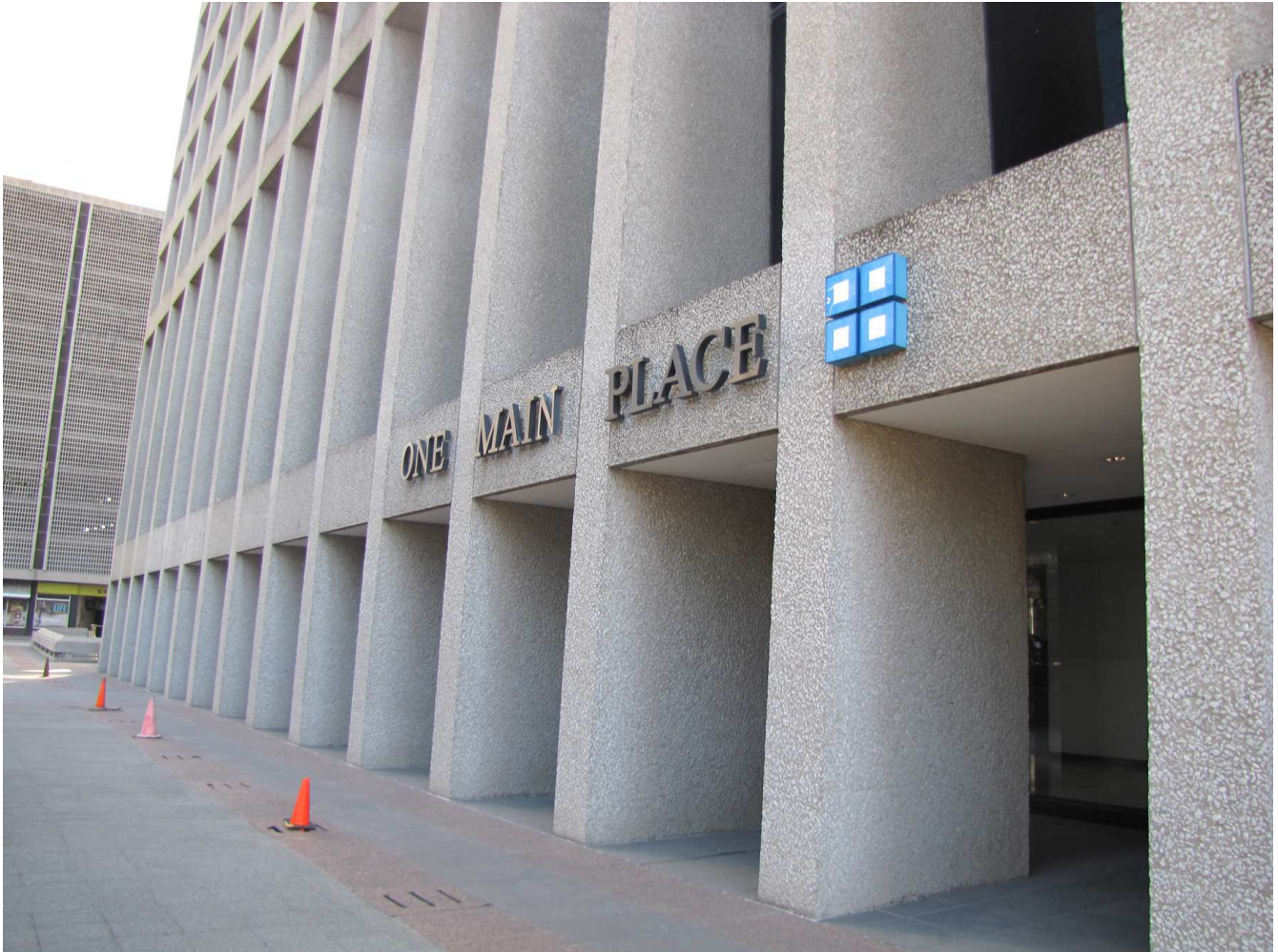
Detail of north facade facing southeast, October 2014
