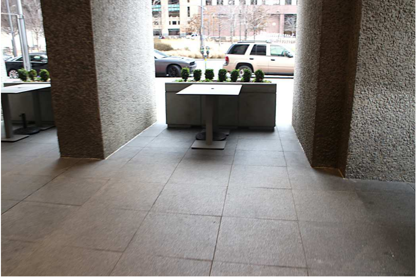
Temporary barrier in south arcade for restaurant tenant, January 2017
