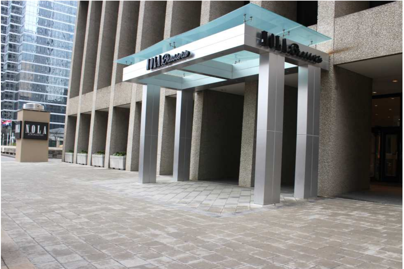
New marquee structure at southwest entry, January 2017
