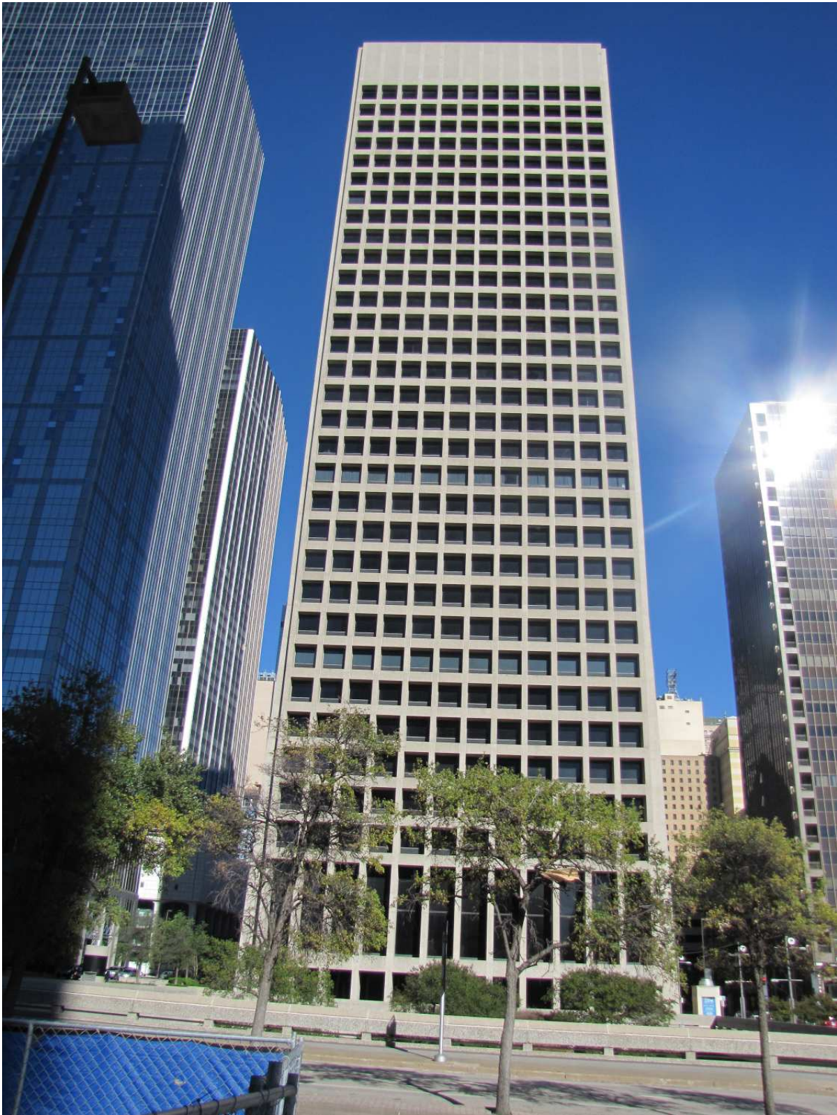
West facade, October 2014
