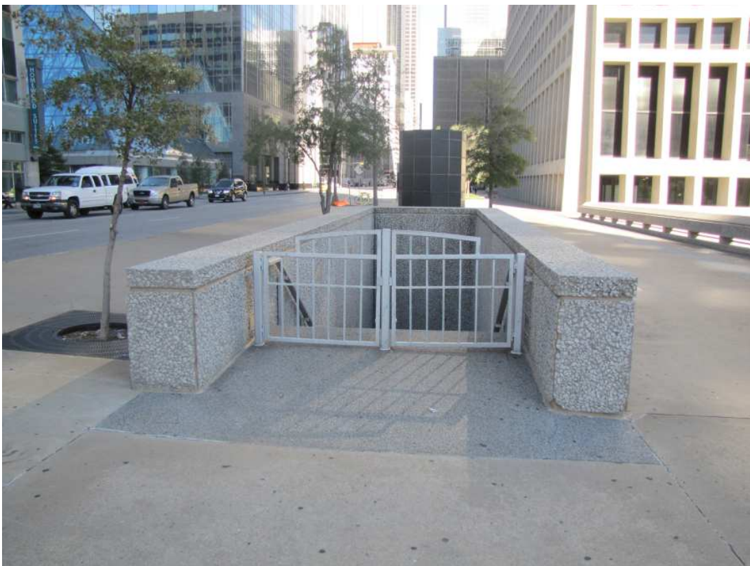
Detail of west sunken-plaza guardrail (top), October 2014 Stair to west sunken-plaza at northwest site (bottom), October 2014
