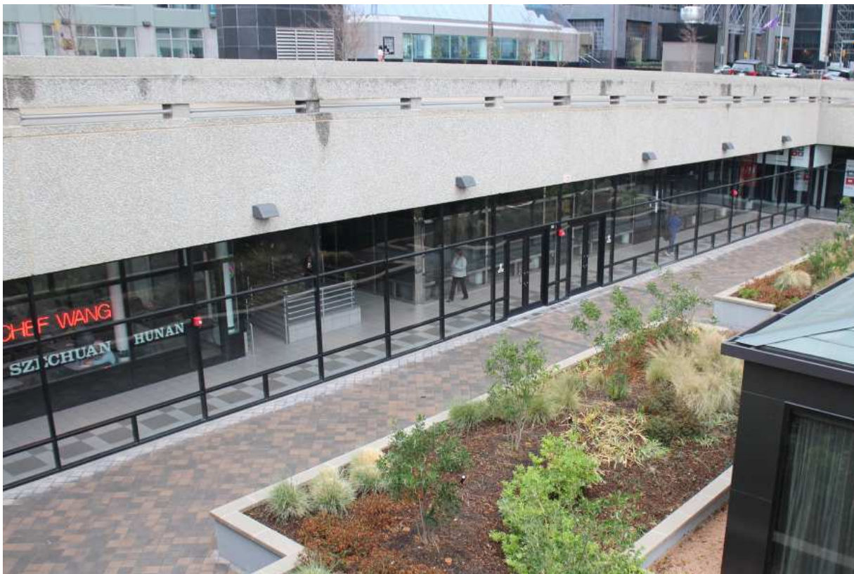
View of rehabilitated west sunken-plaza storefronts, east side (top), and north side (bottom), January 2017
