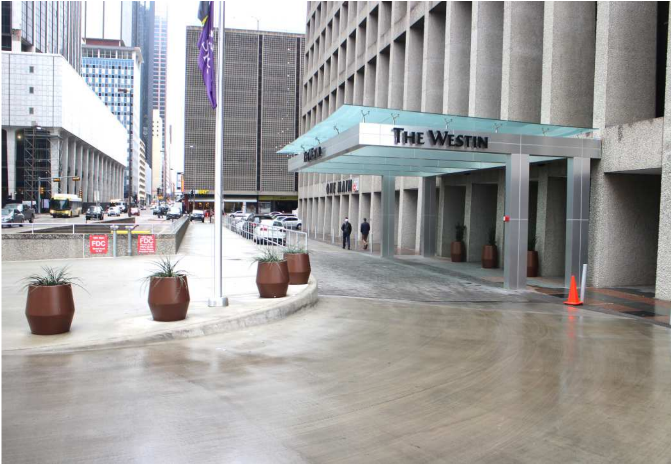
North site from the west showing new porte cochere and drive lane, January 2017
