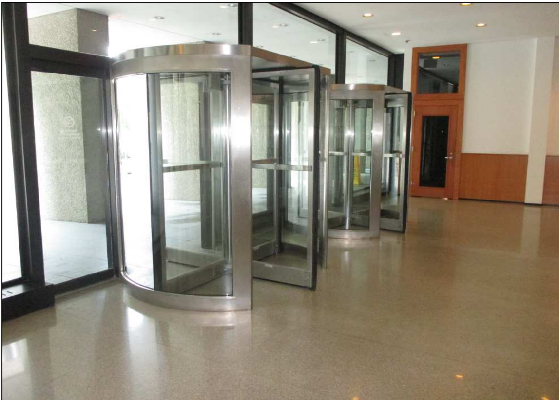
Details of typical revolving door assembly (southwest entry), October 2014
