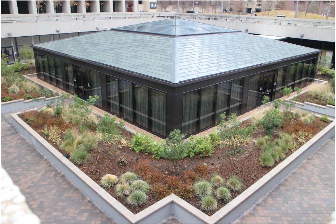
View of west sunken-plaza from street level northwest showing new pavilion and planters, January 2017
