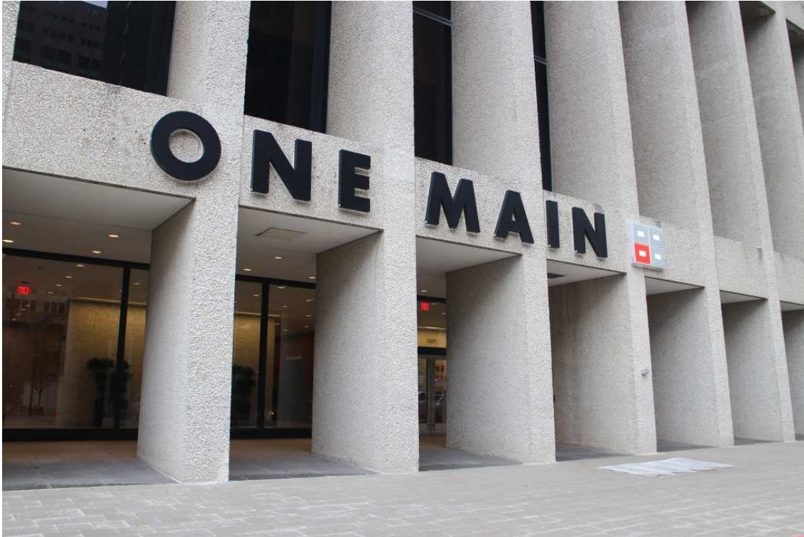
Building identification sign at south arcade (bottom), January 2017
