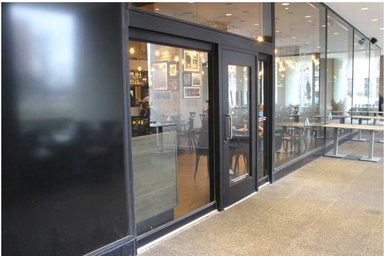
Compatible new entry added for restaurant tenant: at southwest (top) and at west (bottom), January 2017
