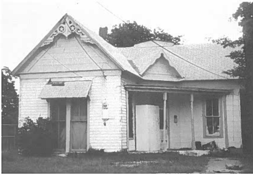
Figure 21. The L-Plan. Before rehabilitation, this house has a roof addition, asbestos siding, one chimney has been removed, another chimney has deteriorated, meter boxes have been added to the building's front.
