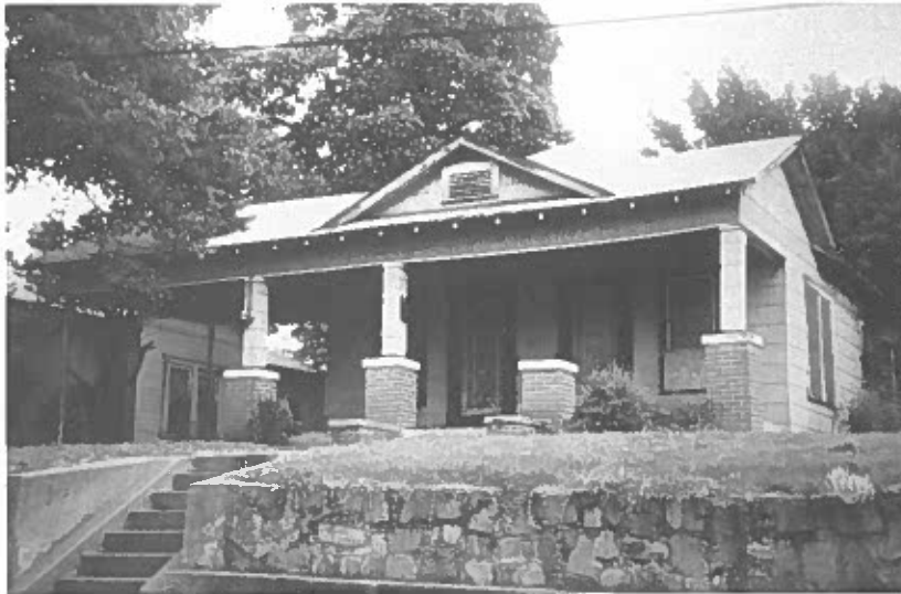
Figure 30. The Craftsman Bungalow. Before rehabilitation, this house has asbestos siding, missing wood boxed column and pipe columns supporting the roof over the driveway.
