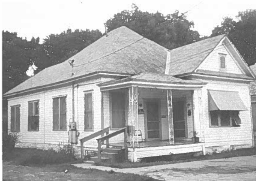
Figure 24. The One-Story Vernacular Queen Anne with gabled front. Before rehabilitation, this house has fabricated metal columns, metal window canopies, missing porch handrail and balusters, and gable window has been converted to a vent.
