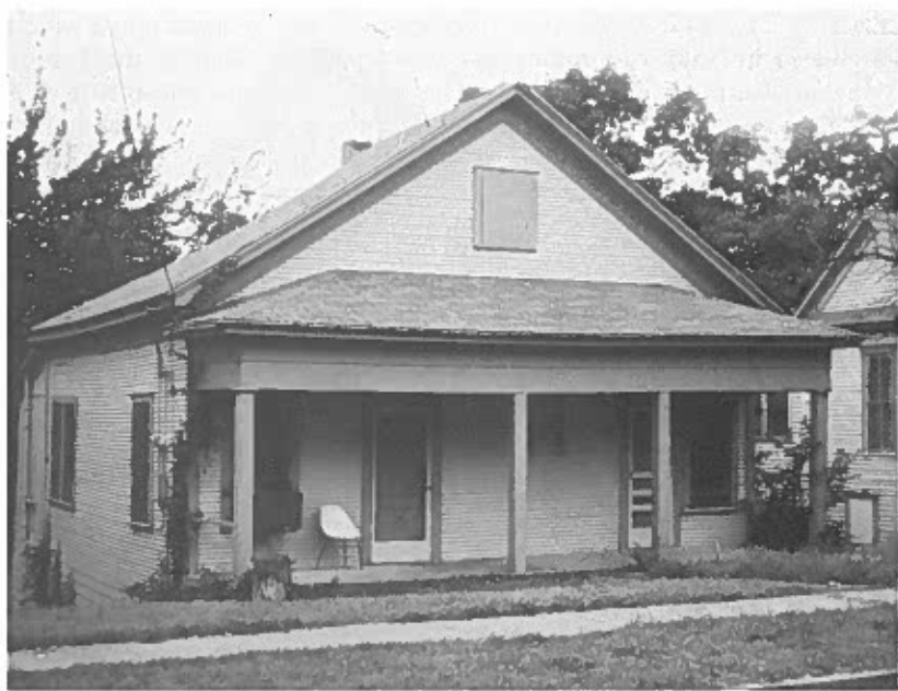
Figure 9. The Double Shotgun. Before rehabilitation, this house has deteriorated brick chimney, boarded up window, and asbestos siding above porch columns.
