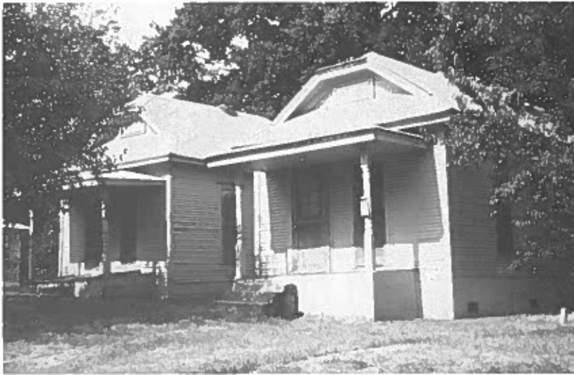
Figure 12. The Camelback. Before rehabilitation, this house has collapsed brick chimneys, no railings or balusters, and modern wood doors.
