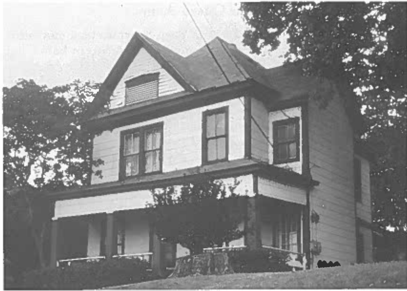
Figure 27. The Two-Story Vernacular Queen Anne with cross-gables. Before rehabilitation, this house has asbestos siding, missing handrail and balusters on porch, attic window converted to vent, windows removed from side elevation, gable end covered by composition shingles, and the addition of modern french doors.
