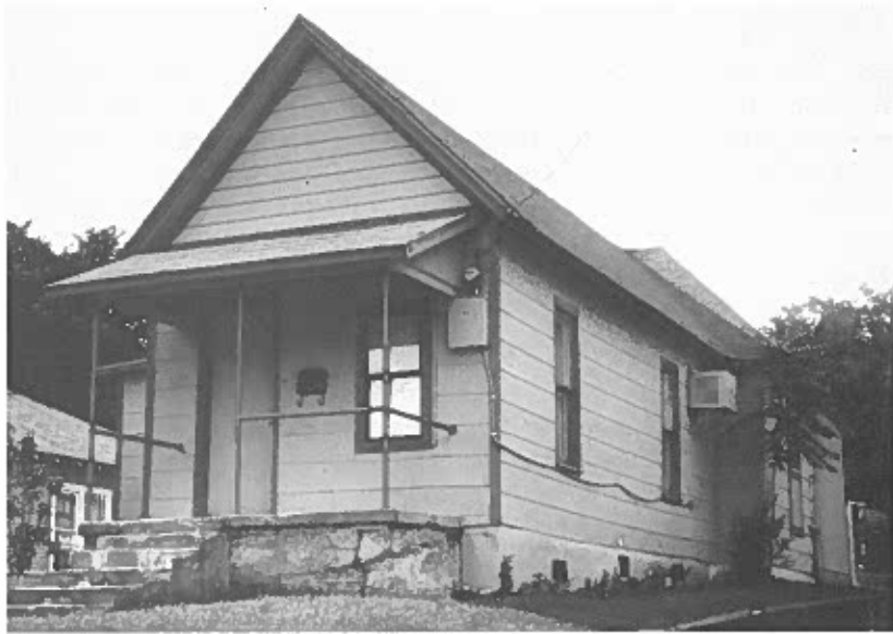
Figure 6. The Shotgun. Before rehabilitation, this house has asbestos siding, aluminum windows, pipe porch columns and rails, meter box on front, and plain solid core door.
