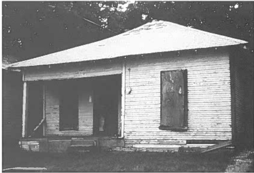
Figure 18. The Pyramidal. Before rehabilitation, this house has unpainted wood siding, boarded up windows, foundation problems, sagging roof and collapsed and missing railing and balusters.
