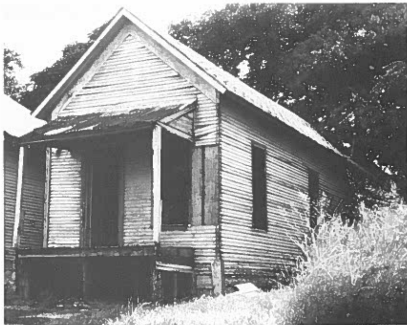
The Tenth Street Shotgun house (c. 1905)
