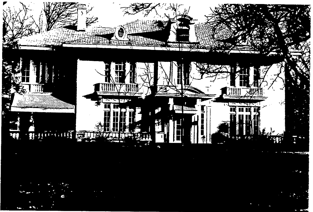
House in the Swiss Avenue Historic District. The facade was restored by the owners. (Stump)
