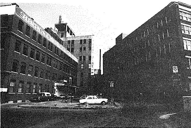
End of Market Street looking north at Munger. Most defined example of exterior space suitable for plaza development.
