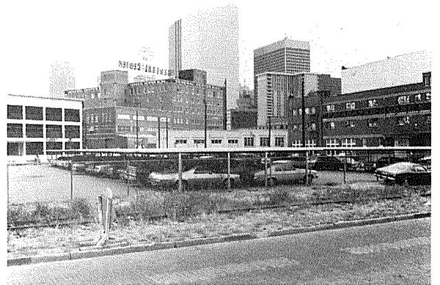
View of parking lot and downtown from Record Street. Curbs badly damaged. Abandoned railroad corridor provides opportunity for parking in the short term.
